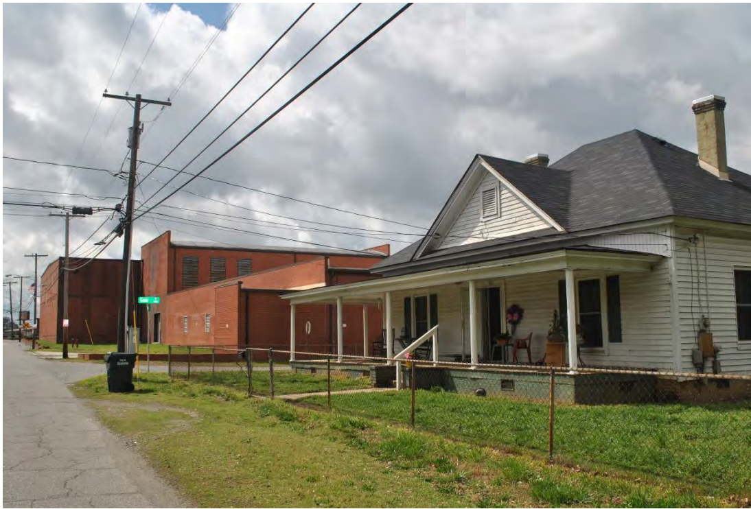
Groves Mill Village, Supervisor's House, 601 Grover Street, Looking South.
