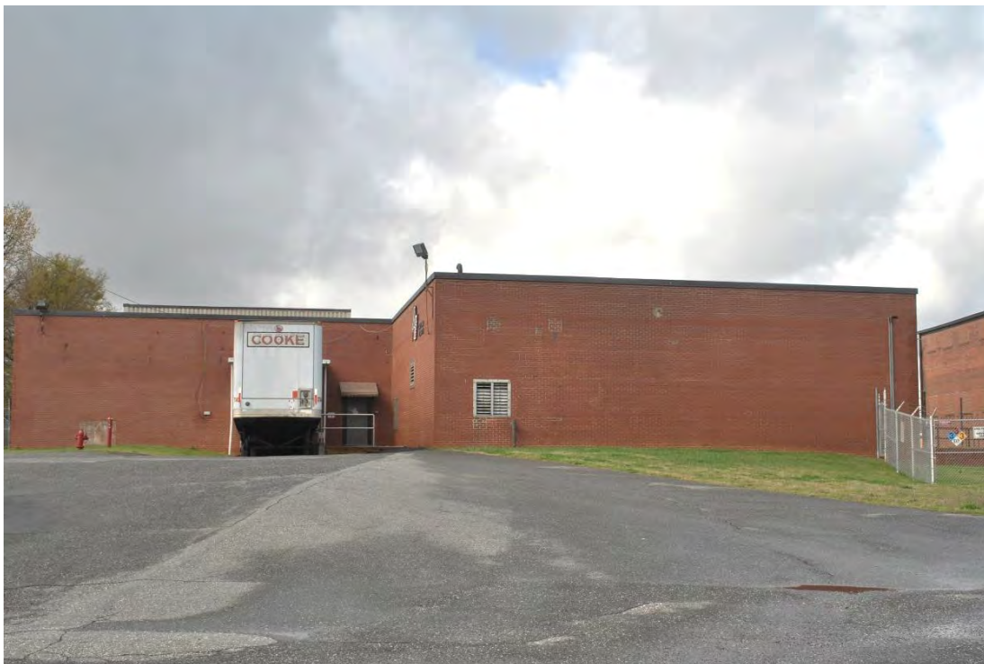
Groves Mills, Mill No. 1, 1959 East Elevation, Looking West from Grover Street
