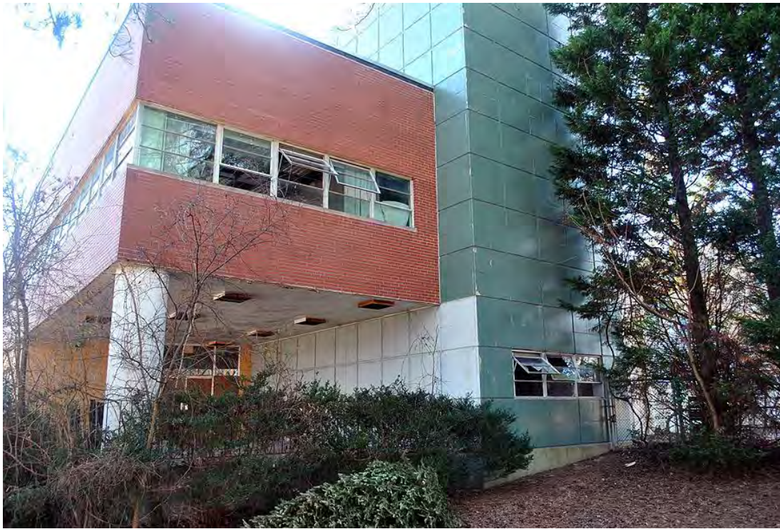
Hinde and Dauch Paper Company Factory, North Bay and Tower, Looking Southwest.
