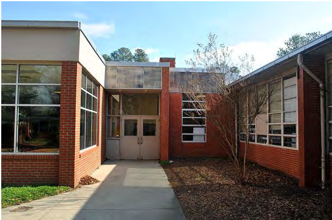
Holbrook High School, 2009 Addition (Left) and East Classroom Building (Right), West Elevation, Looking East.
