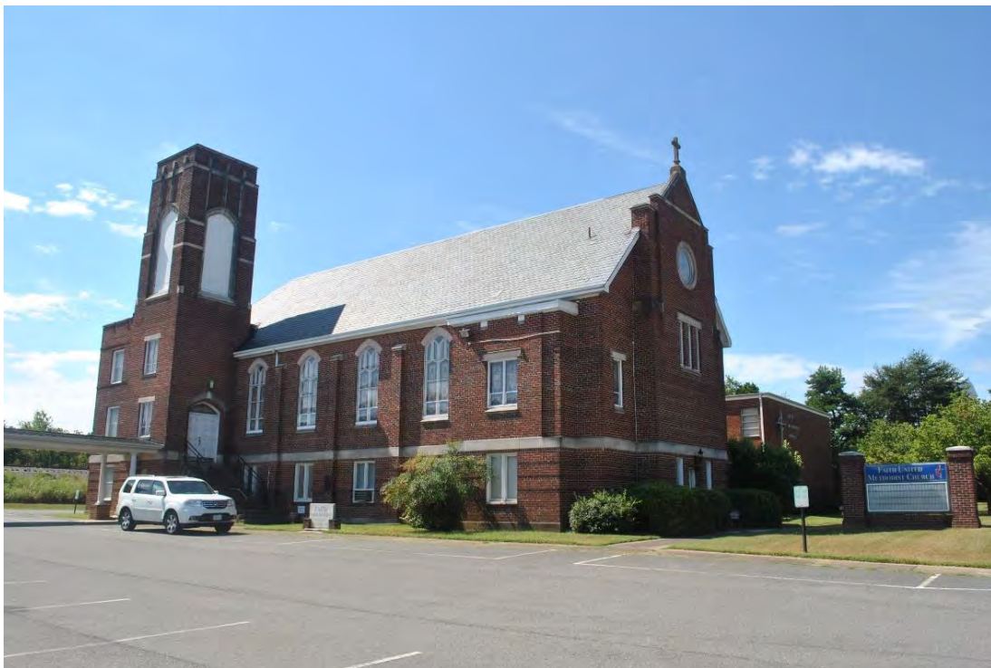
Faith United Methodist Church, Looking Southeast.
