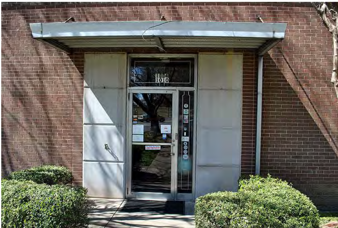
Modena Cotton Mills, Mill No. 1, circa 1965 Front (East) Elevation, Main Entrance.
