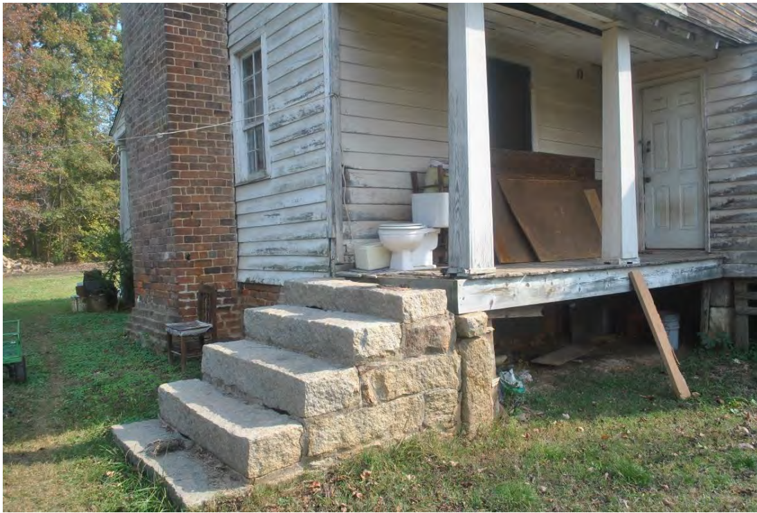
Caleb John Lineberger House, Granite Steps to Rear Porch.
