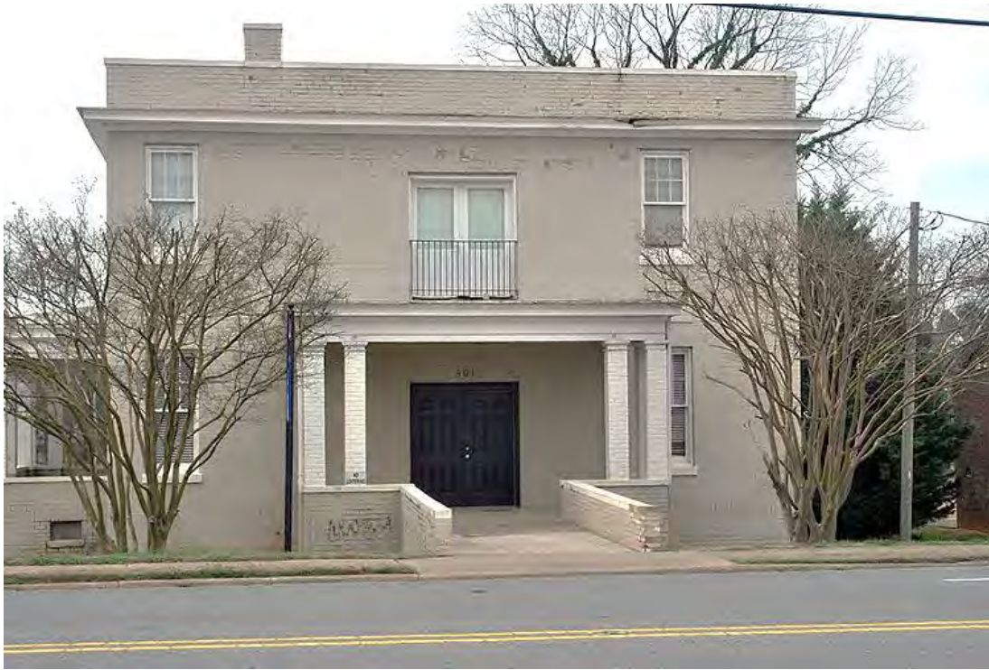
Lowell Teacherage, Side (North) Elevation, Looking South From West First Street.
