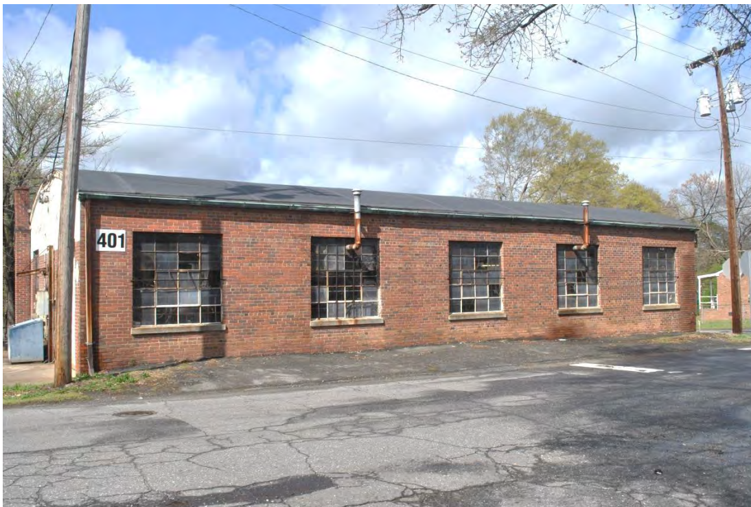
Gastonia Textile Machinery Company, Side (East) Elevation, Looking West.
