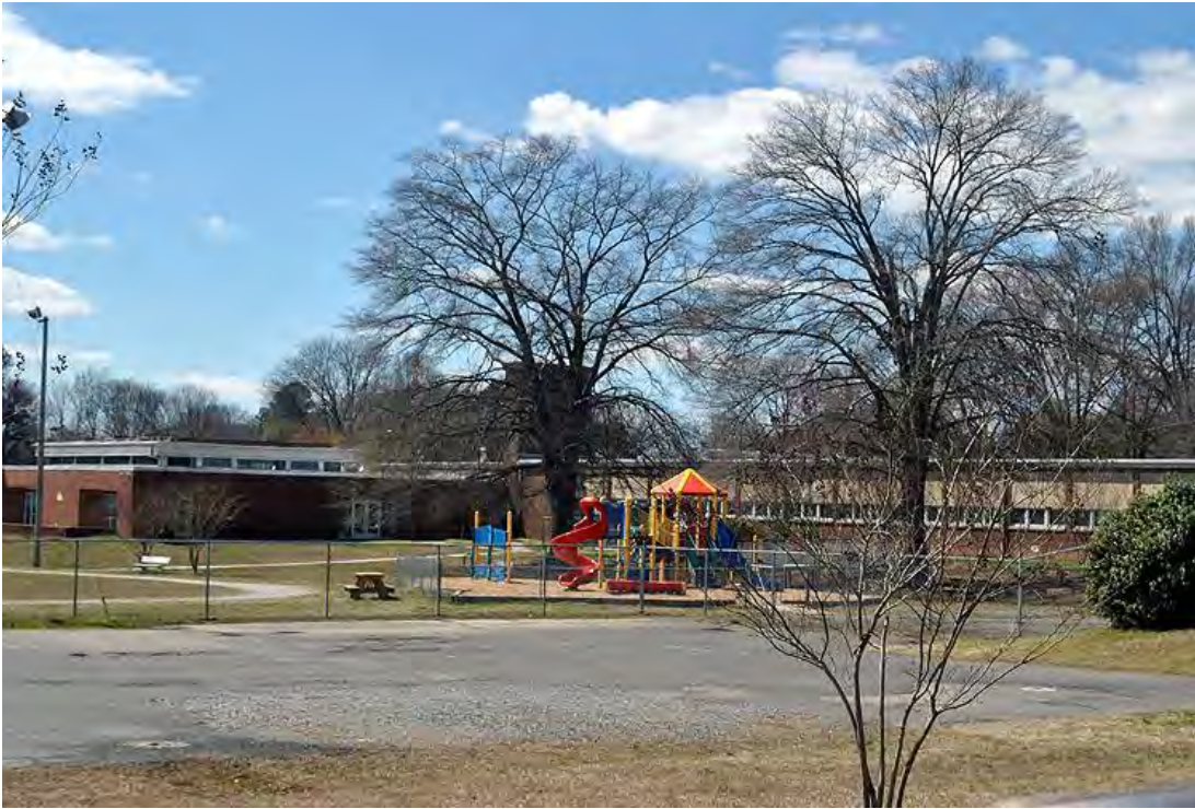
Peedin Elementary School, 1623 Webb Street, Gastonia, Looking West.
