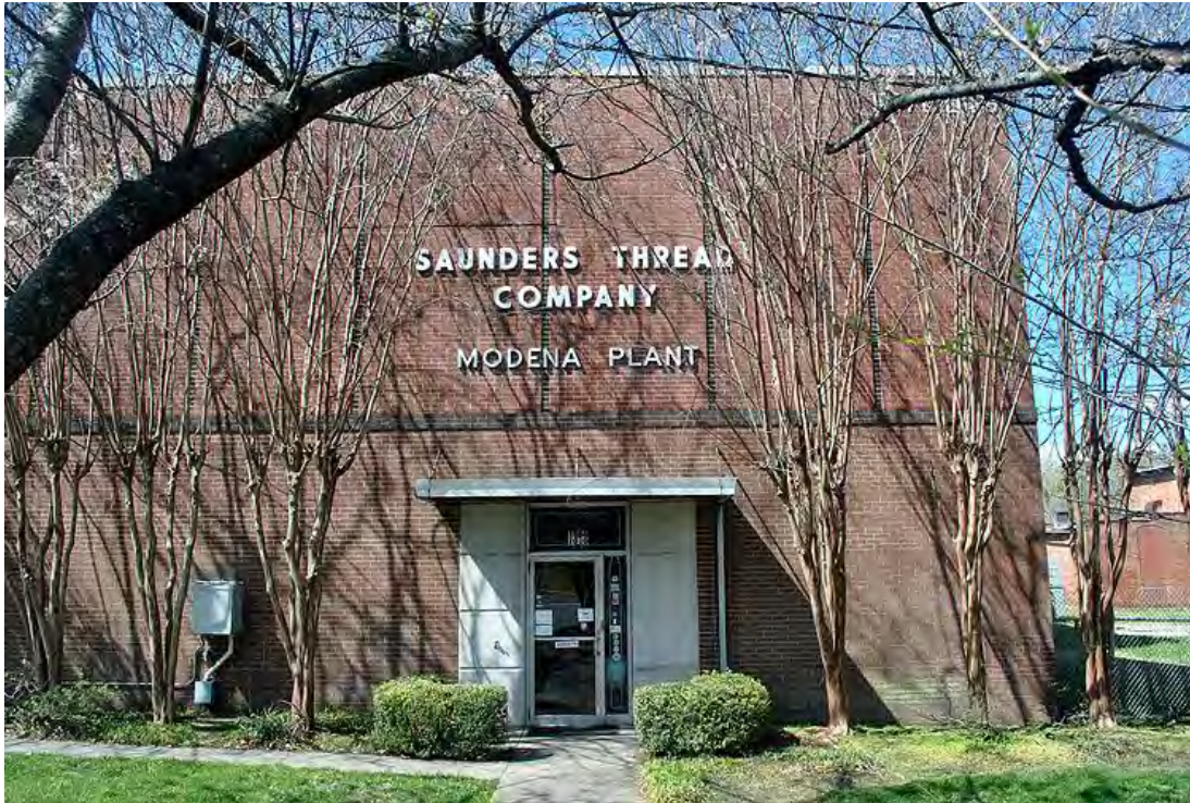
Modena Cotton Mills, Mill No. 1, circa 1965 Front (East) Elevation, Looking West.
