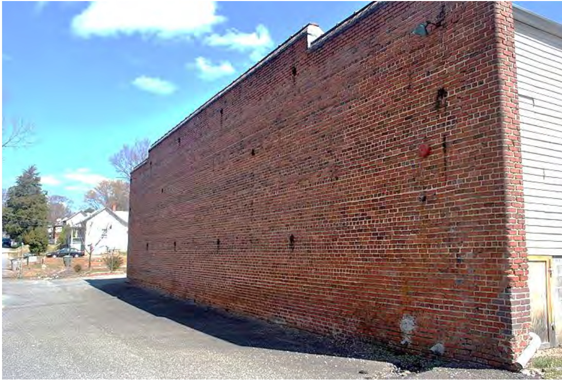
Modena Cotton Mills, Mill No. 2, Cotton Warehouse (1905), West Elevation, Looking North.
