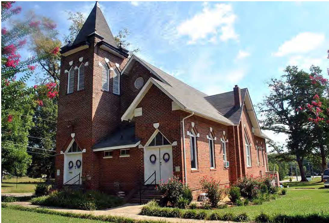
Wrights Chapel A.M.E. Zion Church, Overall View, Looking East.
