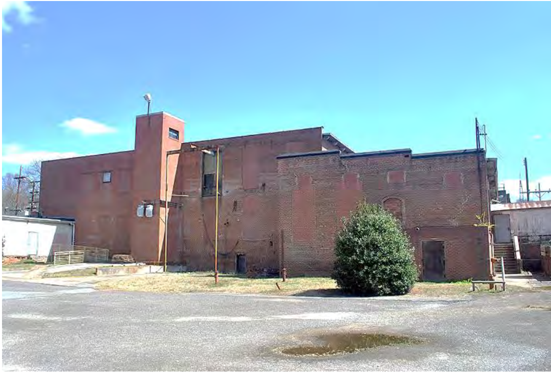
Modena Cotton Mills, Mill No. 2, Rear (West) Elevations, Looking East.
