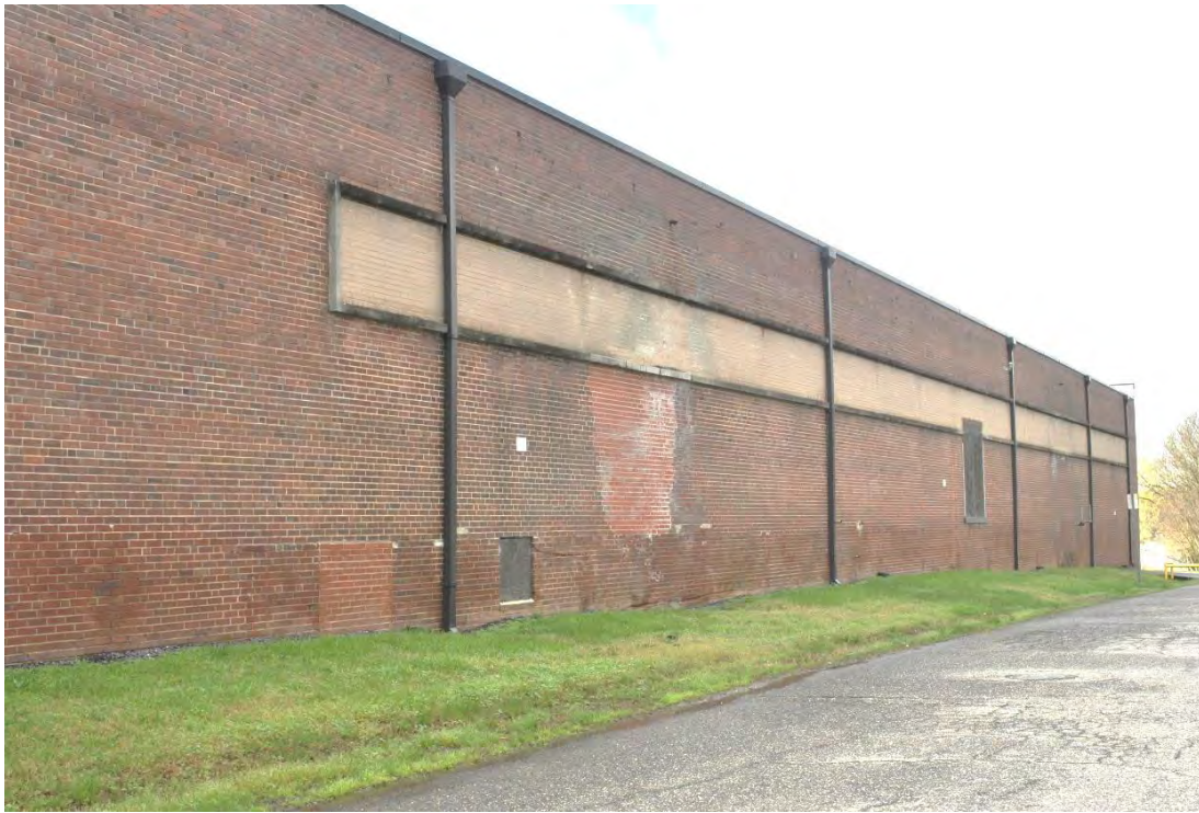
Groves Mills, Mill No. 3, North Elevation along Gum Street, Looking West,
