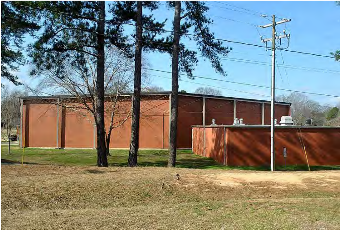
Holbrook High School, Auditorium, Side (East) and Rear (North) Elevations, and Band Room Building, Looking Southwest.
