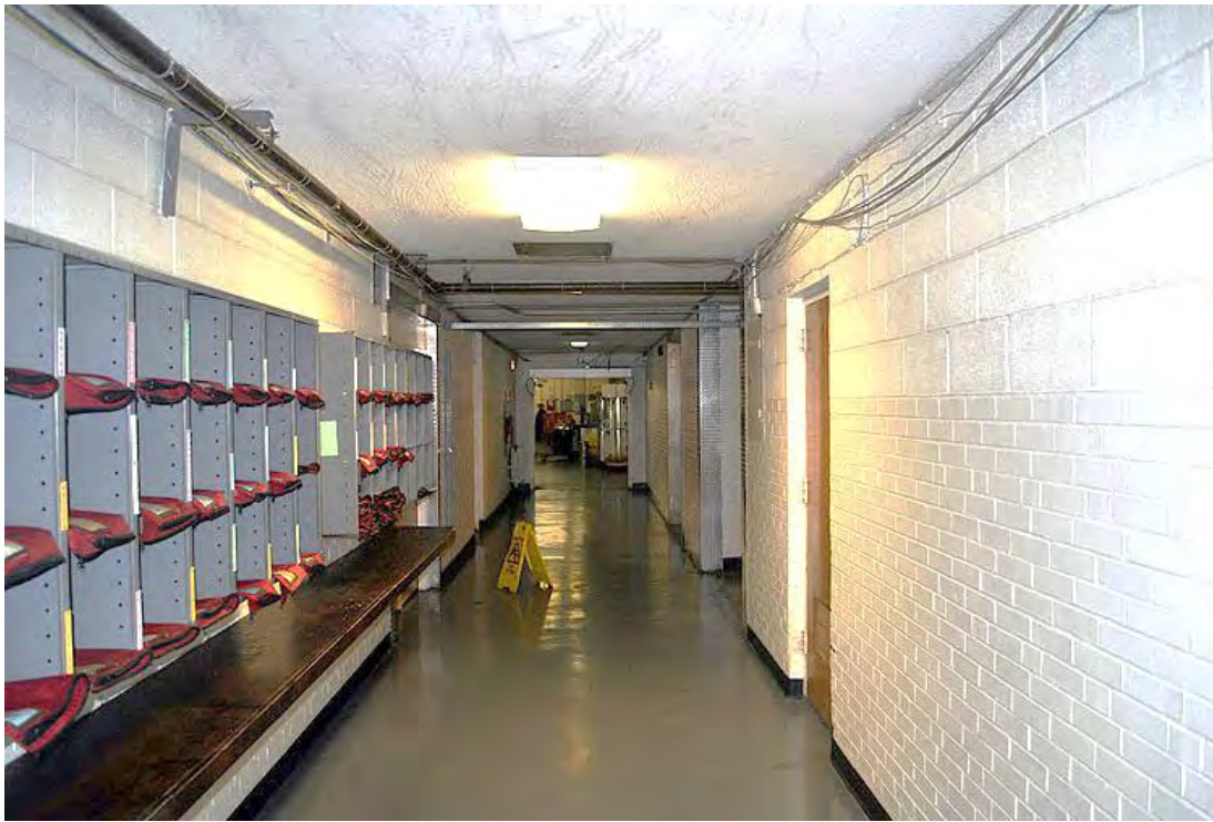
Dora R. Humphrey Elementary School, Interior, Main Corridor, Looking Towards 1988 Addition.
