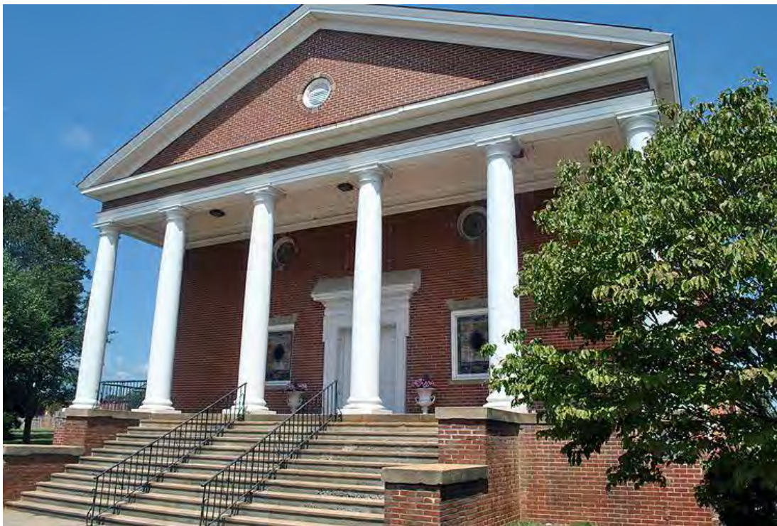
First Baptist Church of Lowell, Front Portico, Looking Northwest.
