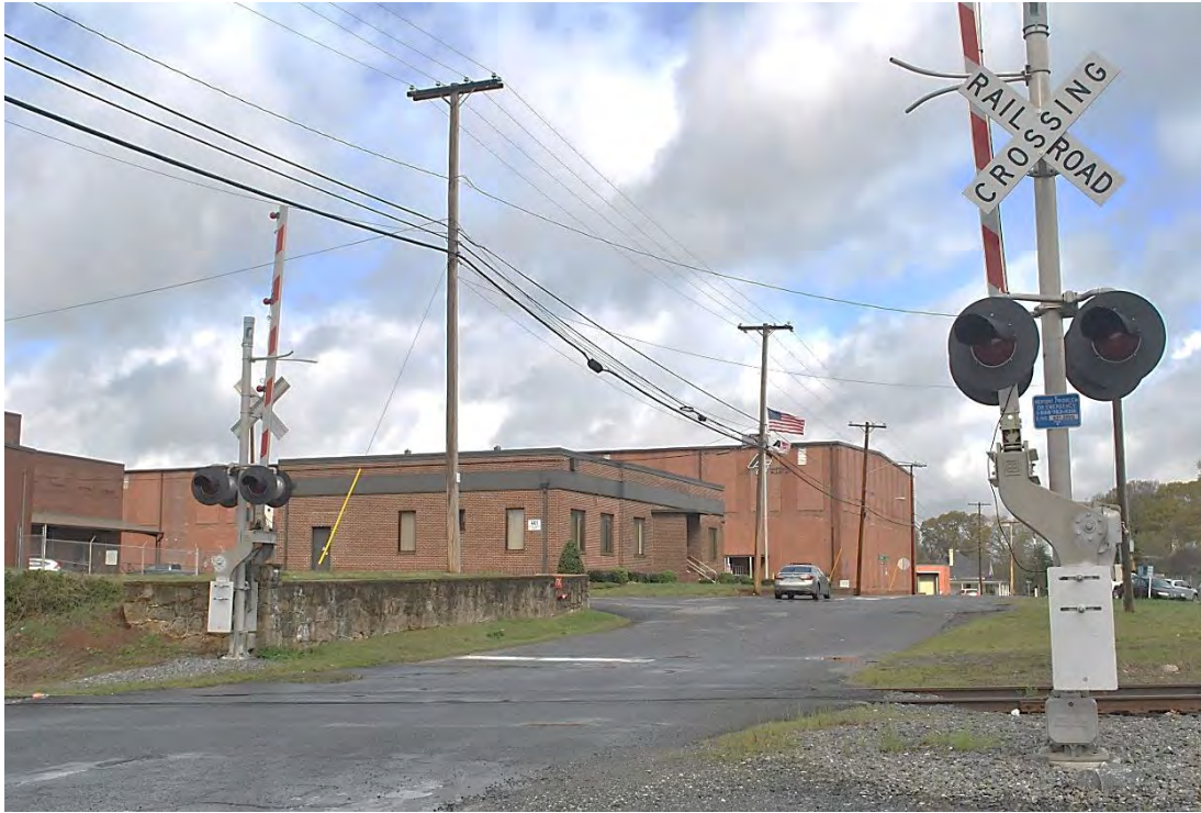
Groves Mills, Mill Office and Mill No. 2, Looking North from P&N Railway.
