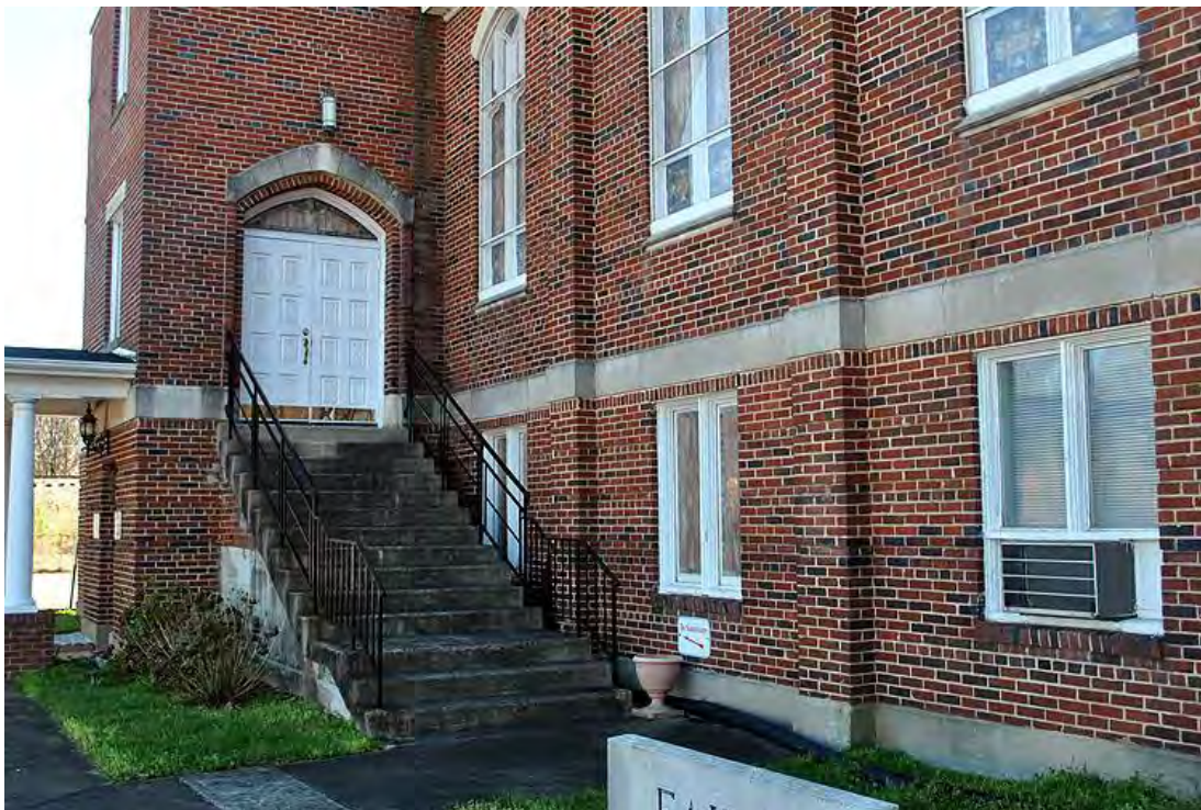
Faith United Methodist Church, Side (North) Elevation, Looking East.
