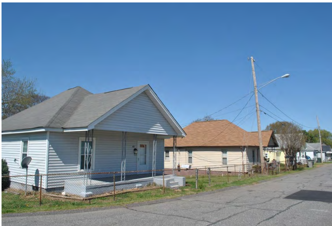
Groves Mill Village, 400 Block of Apple Street, Looking North.
