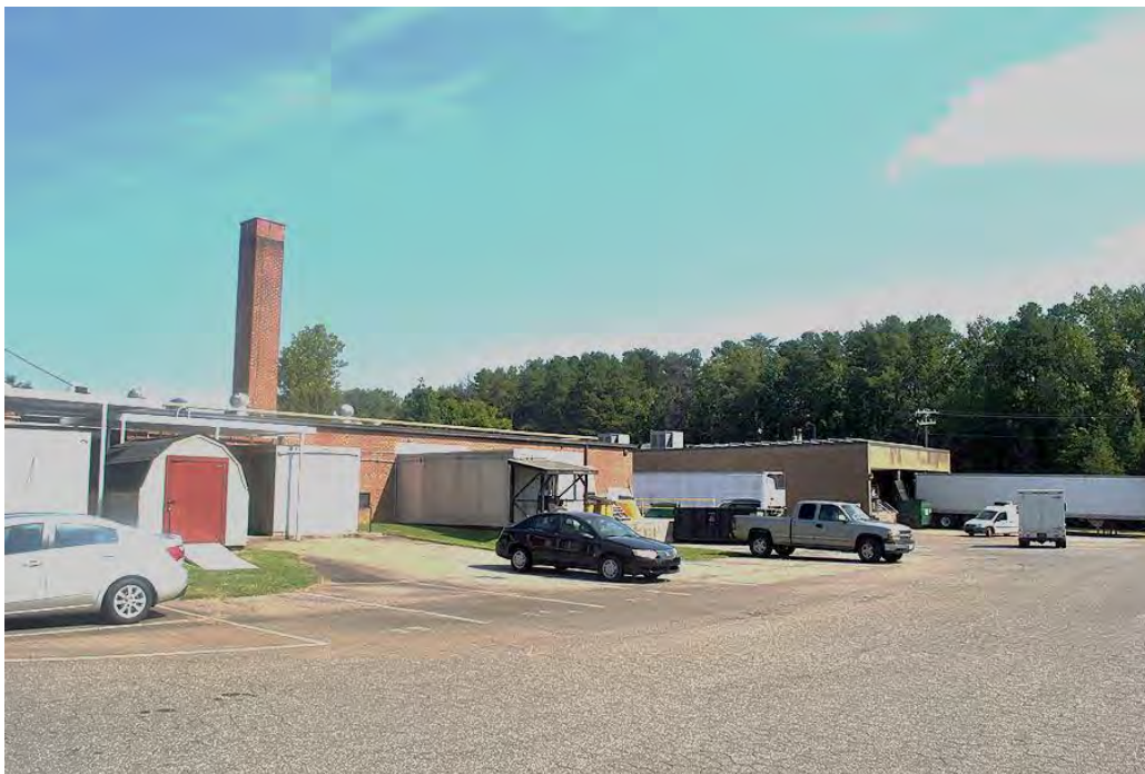
Dora R. Humphrey Elementary School, South (Rear) Elevation and 1988 Addition, Looking North.
