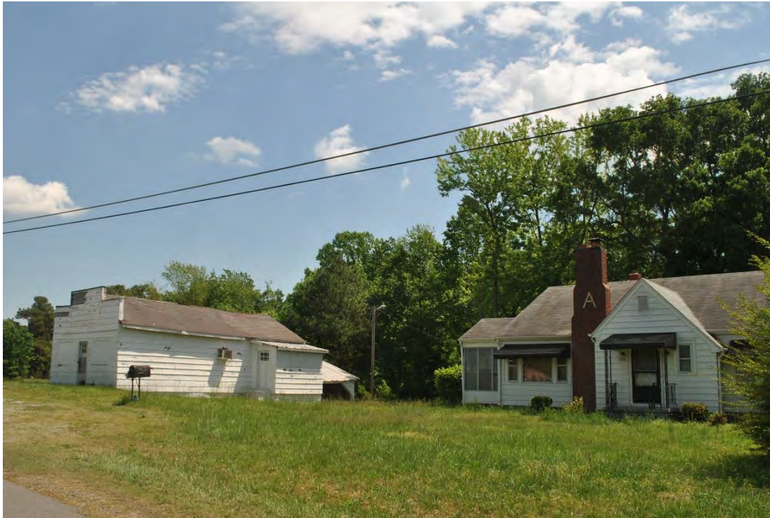
C.V. Alexander Grocery, 209 C.V. Alexander Drive, Bessemer City Vicinity, Looking East.
