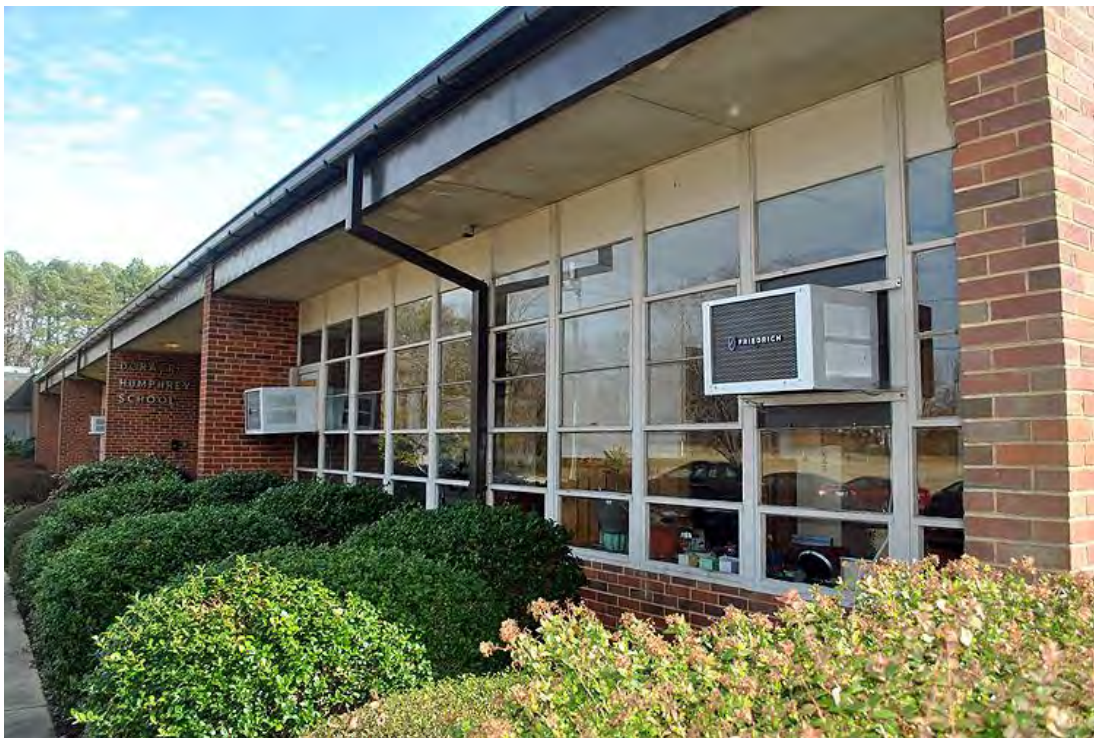
Dora R. Humphrey Elementary School, Façade (North Elevation), Looking East.
