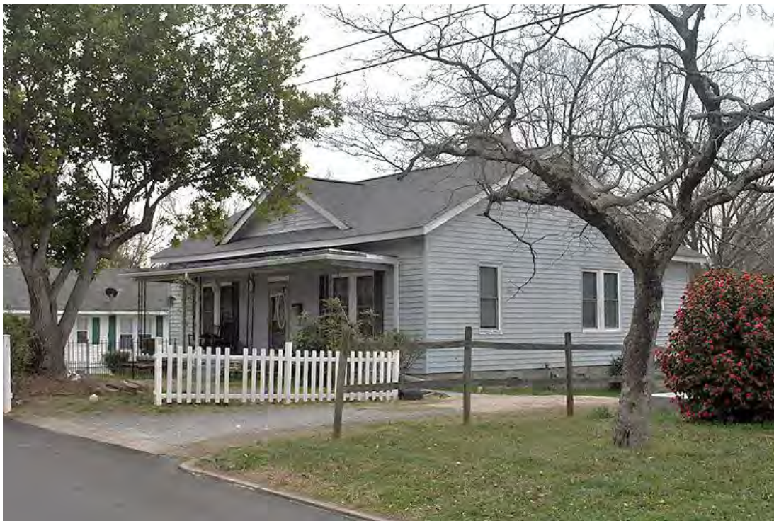
Reid Rosenthal School Teacherage, 223 Cedar Street, Belmont, Looking Southeast.
