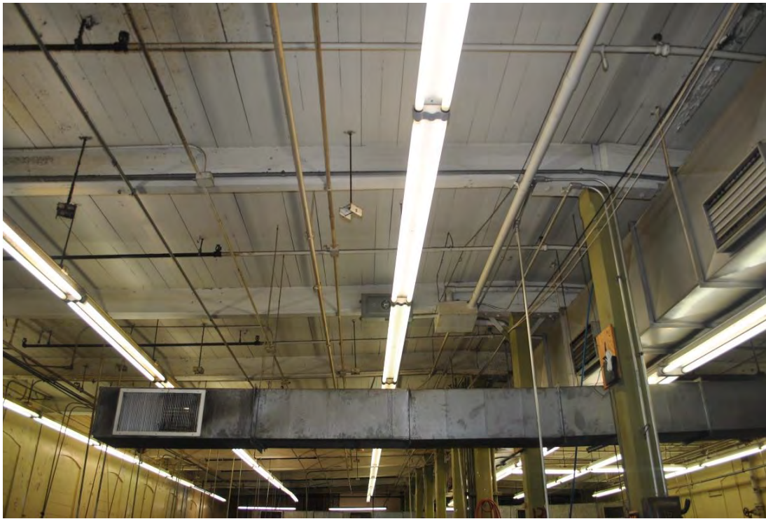
Modena Cotton Mills, Mill No. 1, Interior, Rear Wing (1896), Manufacturing Room, Ceiling,
