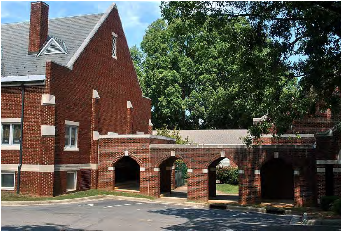
Lutheran Chapel and Cemetery, Rear (East) Elevation and Breezeway, Looking North.
