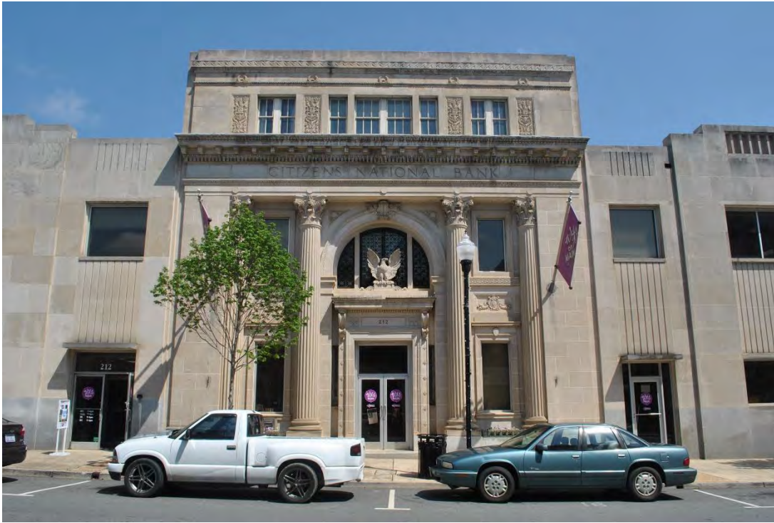
First Citizen's Bank, 210-220 West Main Avenue, Gastonia, Looking North.
