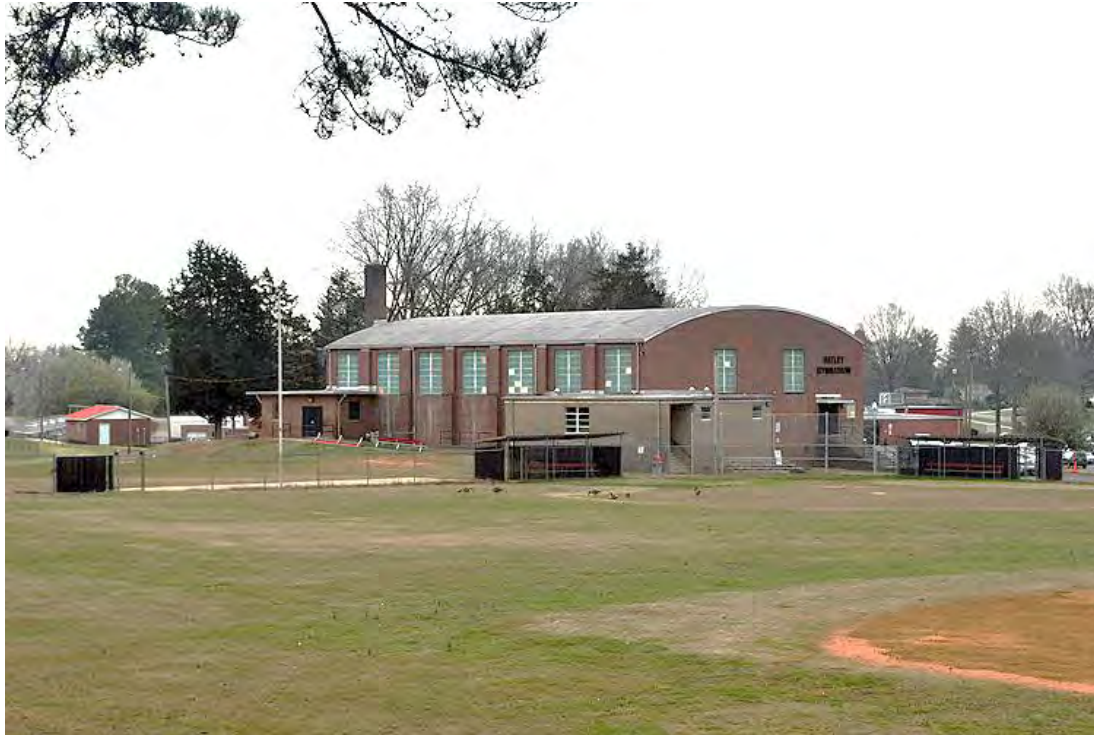
Holbrook High School, Gymnasium, North and West Elevations, Looking Southeast from Athletic Field.
