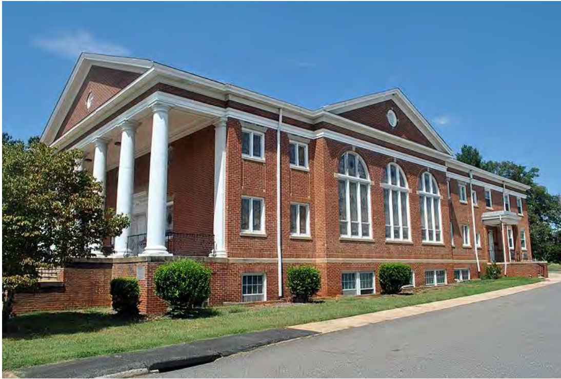
First Baptist Church of Lowell, Front (South) and Side (East) Elevations, Looking Northwest.
