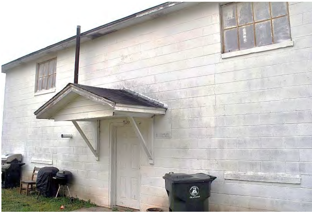
Hiram Masonic Lodge No. 22, Façade (North Elevation), Looking Southeast.
