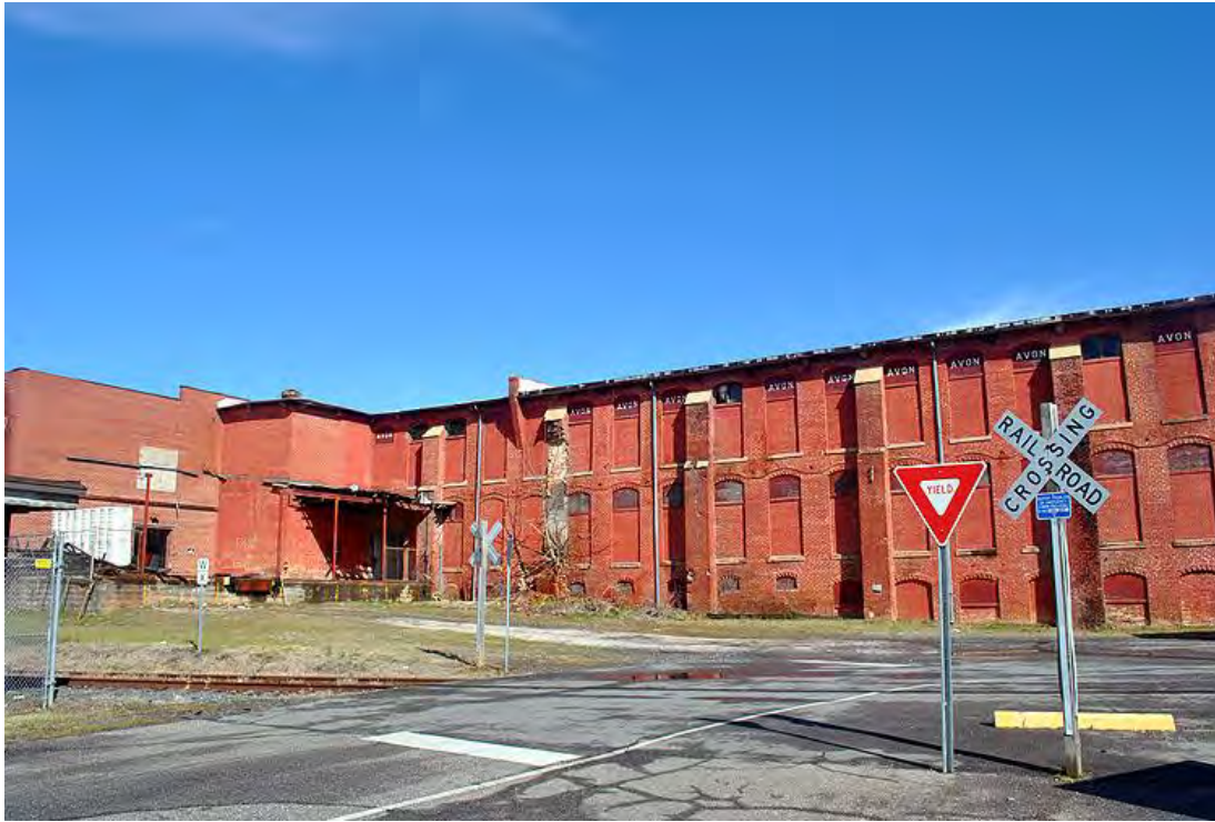
Avon Mills, 601 East Main Avenue, Gastonia, Looking North.
