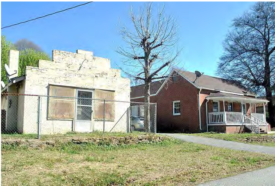
Modena Mill Village, 410-412 North Pine Street, Looking Northeast.
