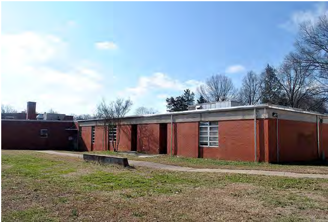
Holbrook High School, 1975 Addition to East Classroom Building, North Elevation, Looking Southwest.
