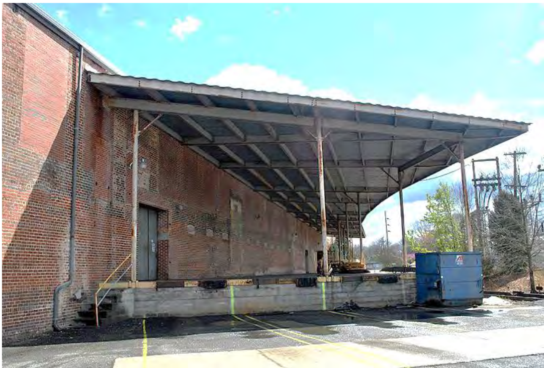
Seminole Mills, 1029 South Marietta Street, Gastonia, Loading Dock, Looking East.
