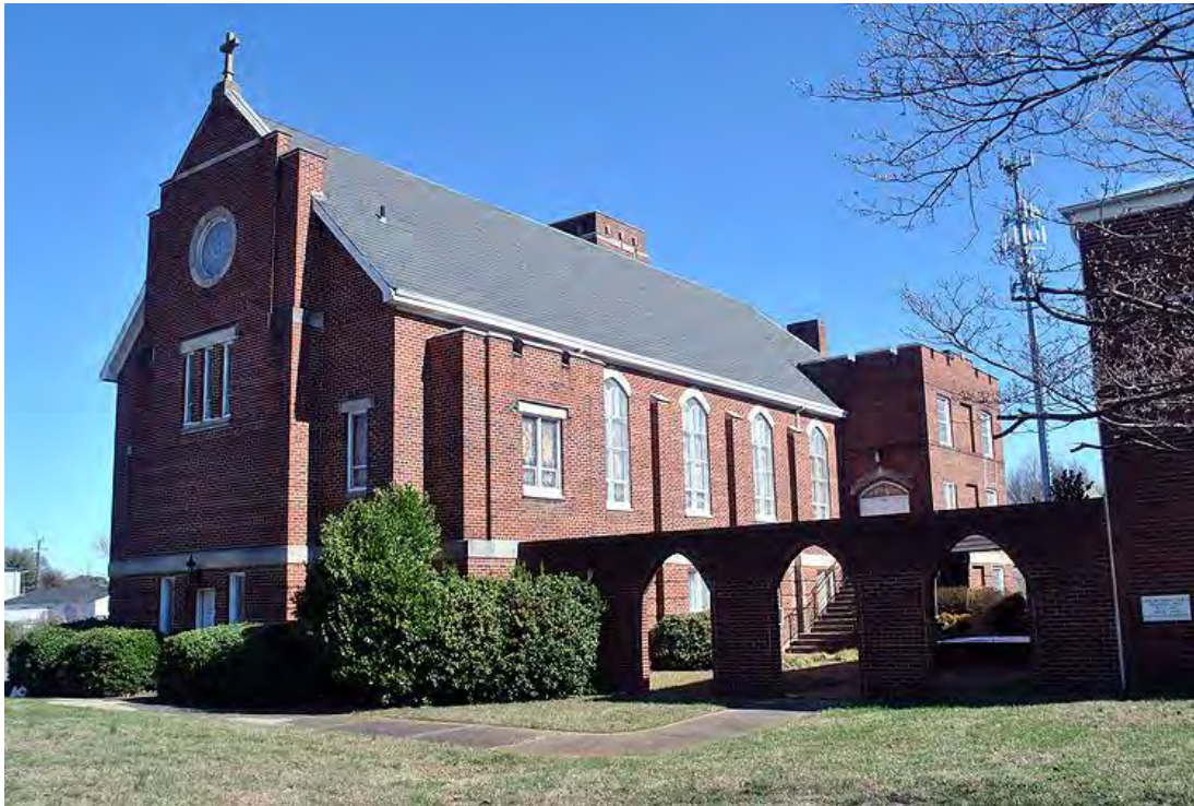
Faith United Methodist Church, Looking Northeast.
