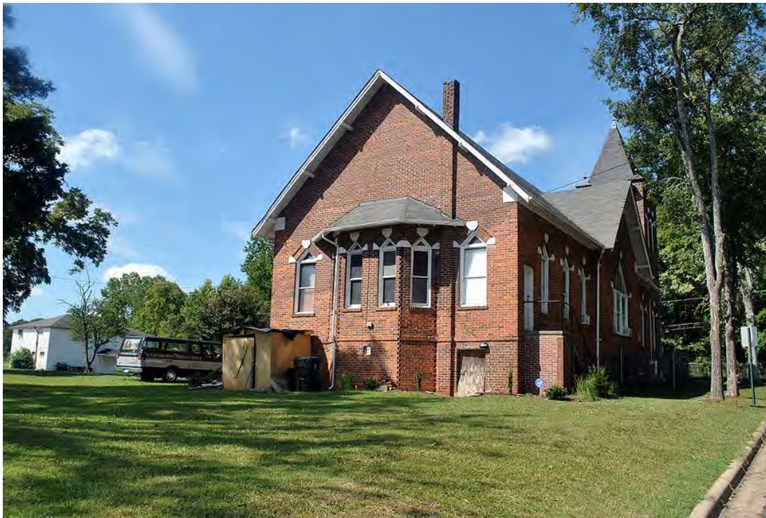
Wrights Chapel A.M.E. Zion Church, Rear (East) Elevation, Looking West.
