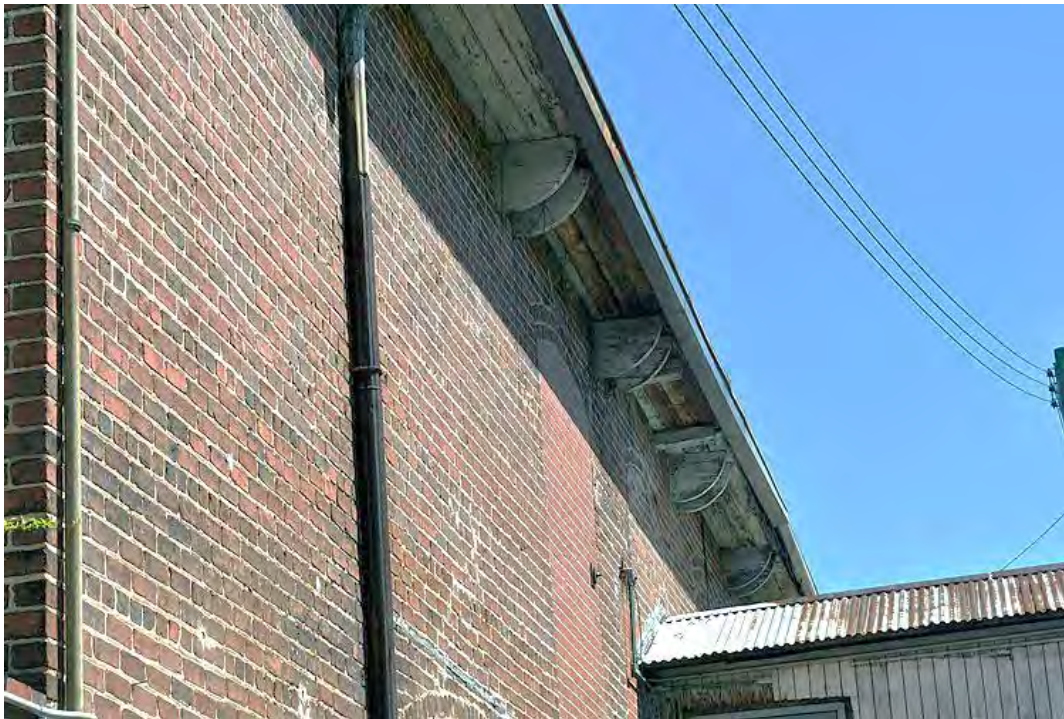
Modena Cotton Mills, Mill No. 2, Side (South) Elevation (1905), Detail, Looking East.
