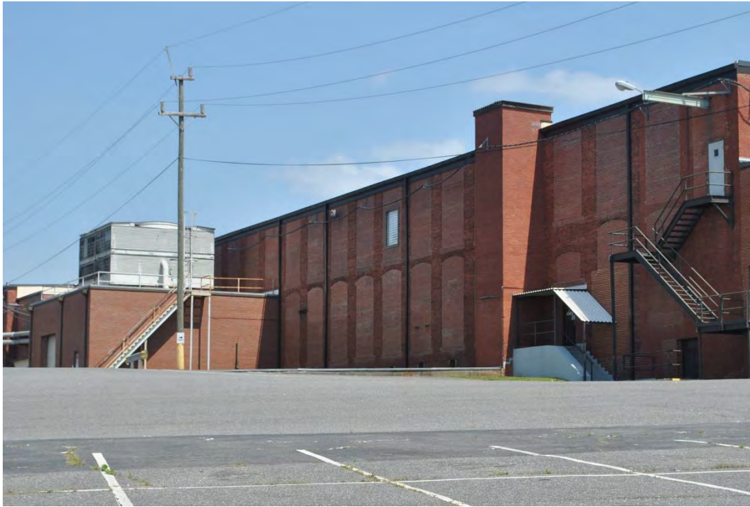
Groves Mills, Mill No. 1, North Elevation, Looking East from Apple Street.
