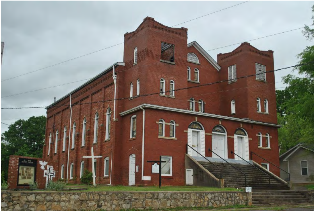
Saint Paul's Baptist Church, 418 North Oakland Street, Gastonia, Looking East.
