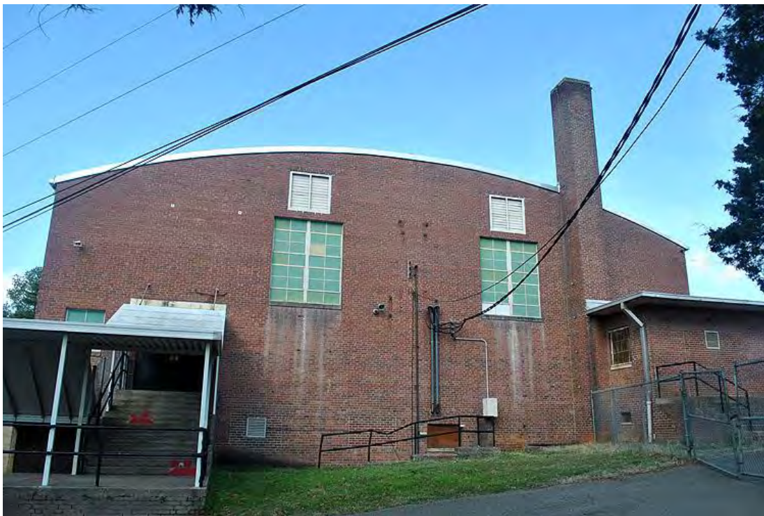
Holbrook High School, Gymnasium, East Elevation, Looking West.
