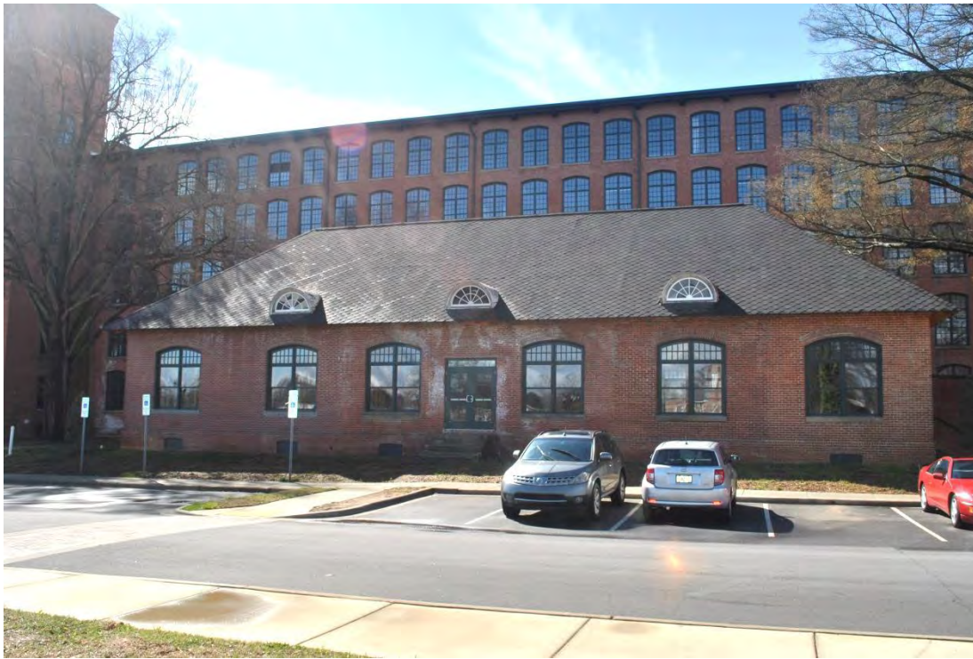
Loray Mill Office, 300 South Firestone Street, Gastonia, Looking South.
