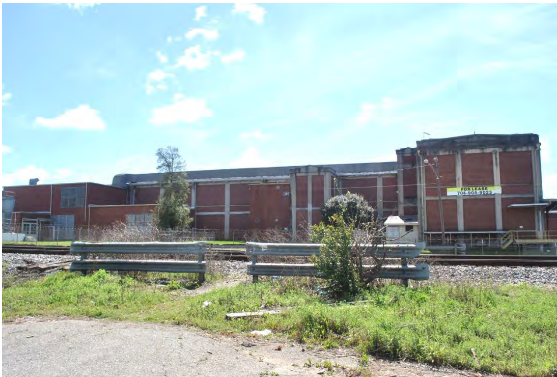
Flint Manufacturing Company, Mill No. 2, Rear (North) Elevation, Looking South.
