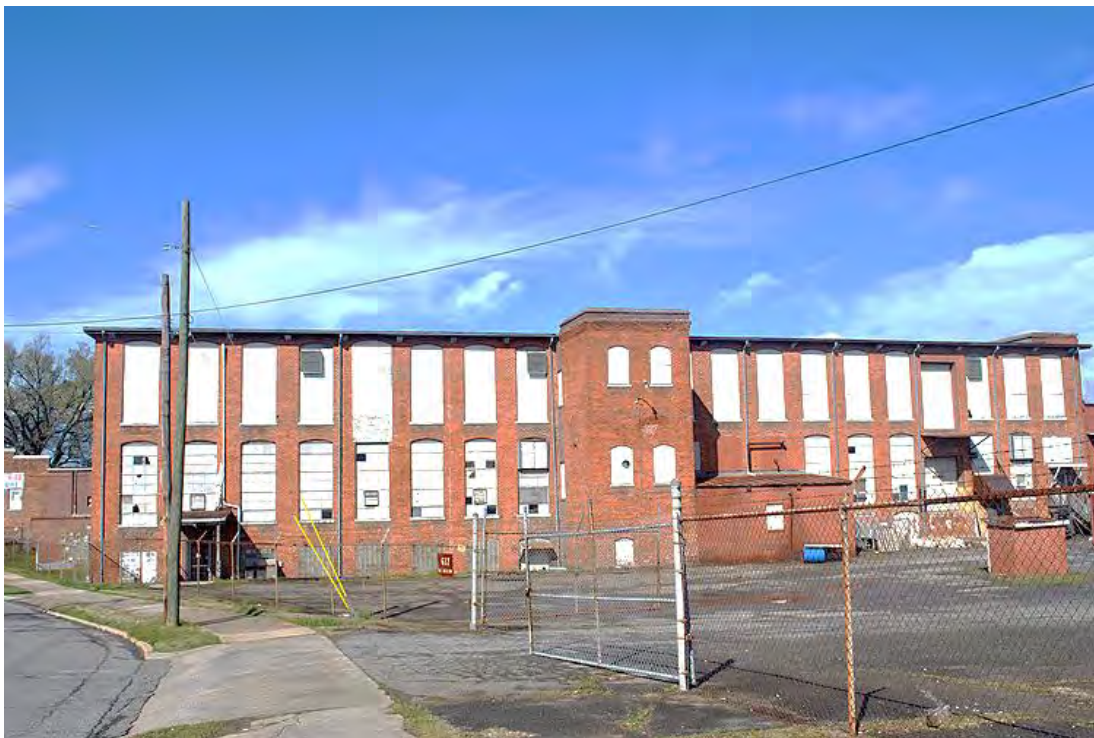
Trenton Mills, 612 West Main Avenue, Gastonia, Looking West.
