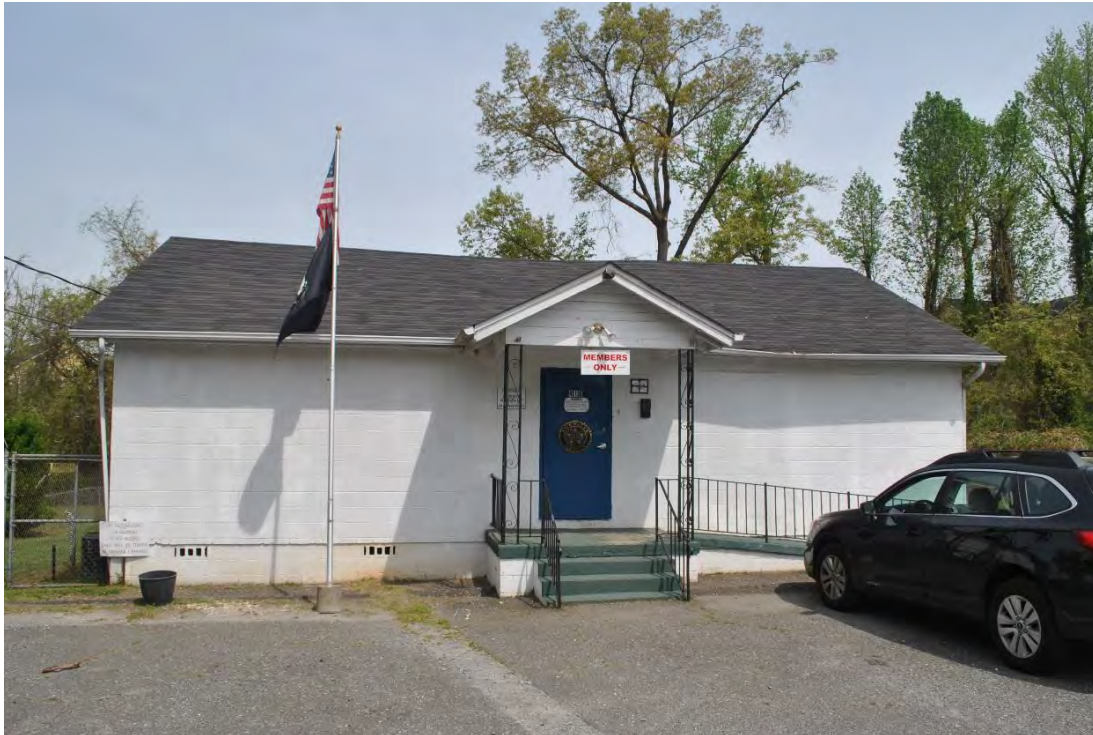
American Legion Hall, Post 180, 418 Lincoln Street, Belmont, Looking North.
