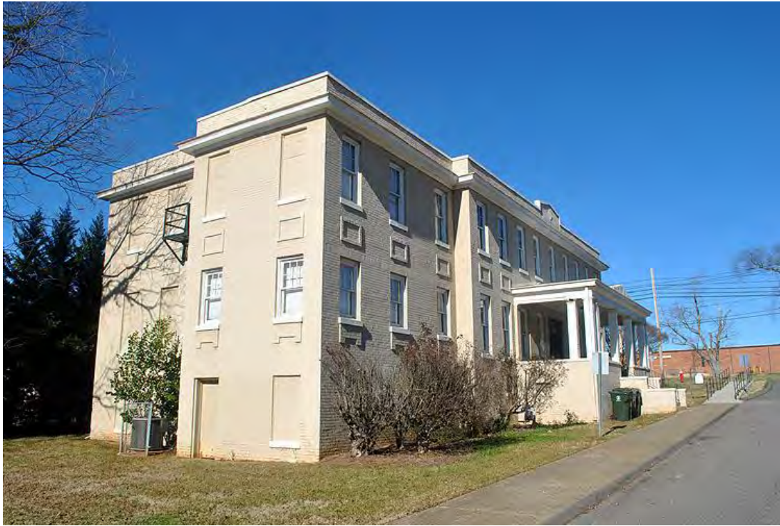
Lowell Teacherage, Side (South) Elevation and Façade, Looking North (Peerless Mill in Background).
