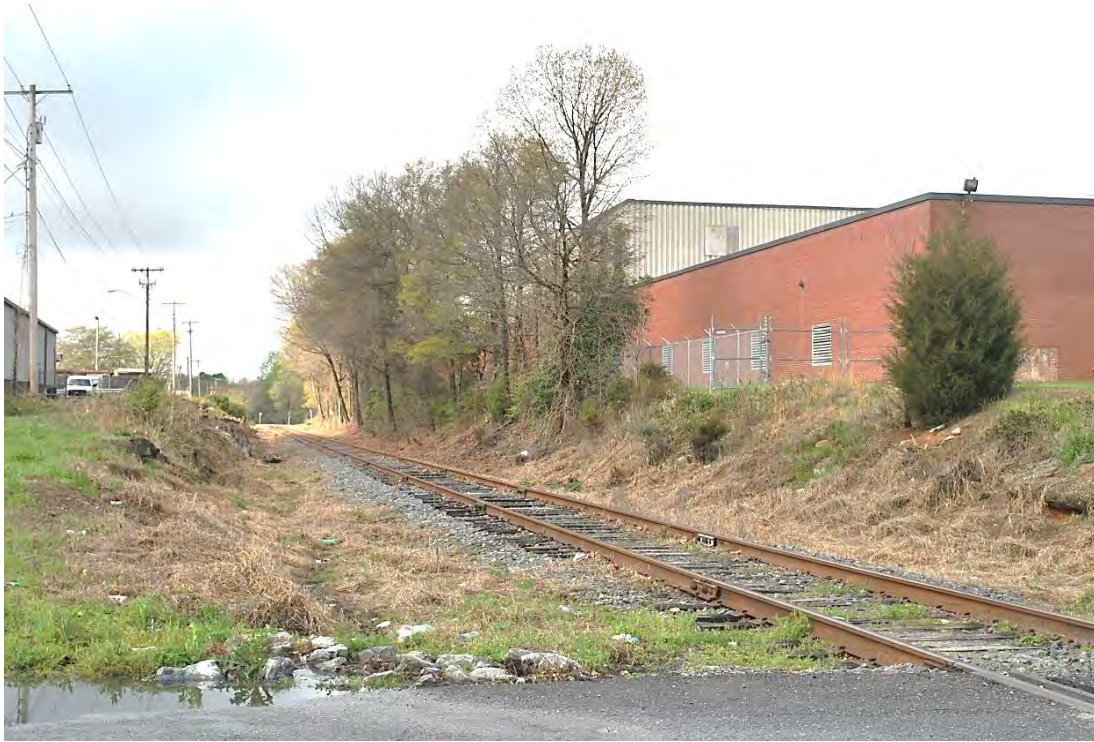
Groves Mills, Mill No. 1, South Elevation, Looking West Along P&N Railway.
