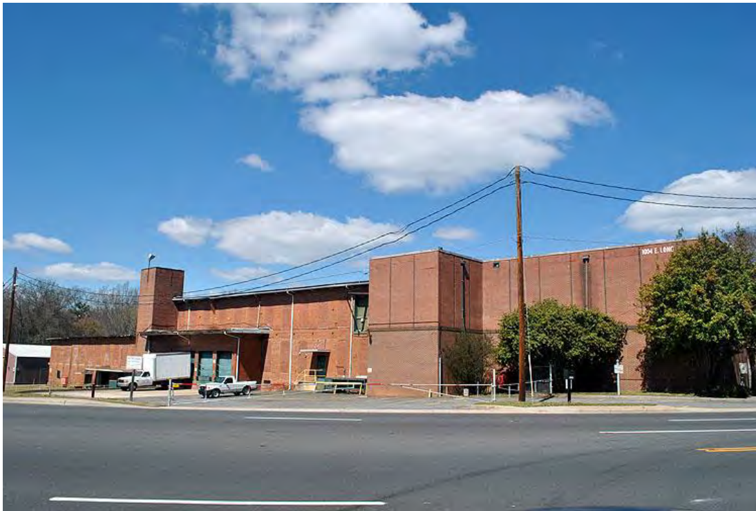
Modena Cotton Mills, Mill No. 1, Side (South) Elevation, Looking Northwest From East Long Avenue.
