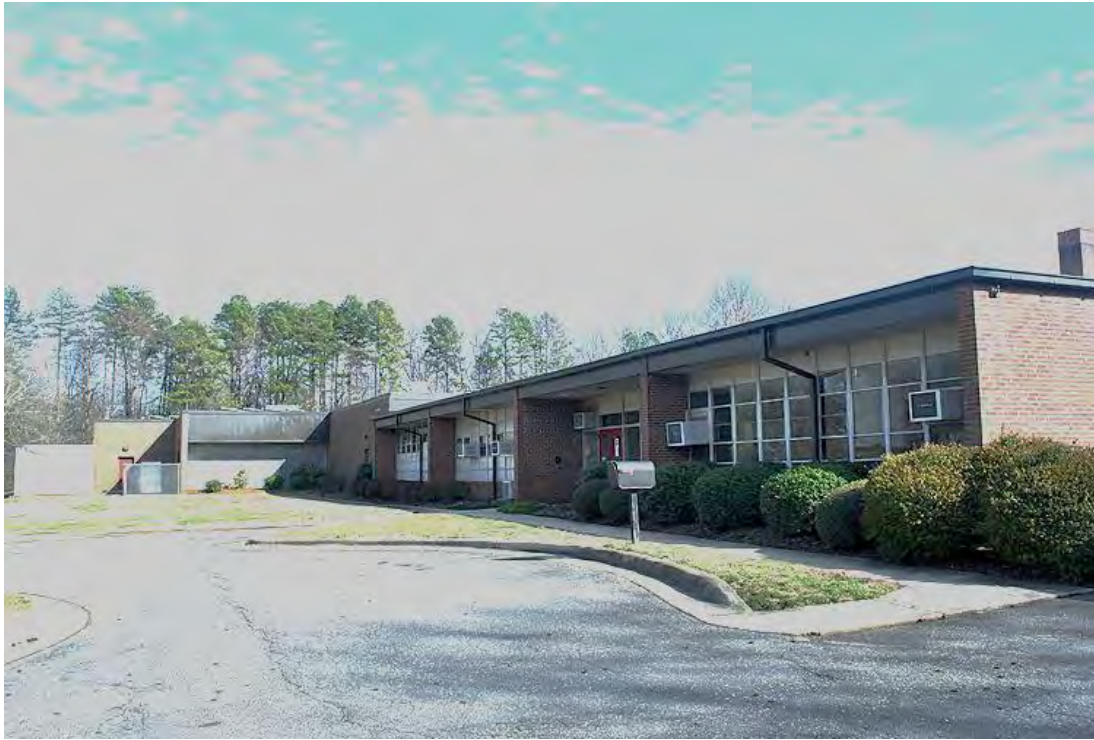
Dora R. Humphrey Elementary School, Façade (North Elevation), Looking East towards 1988 Addition.
