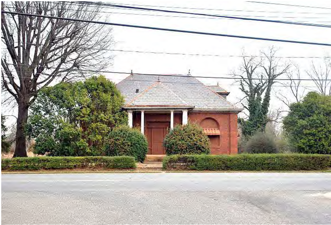
Lowell Cotton Mills, Mill Office, Overall View, Looking North.
