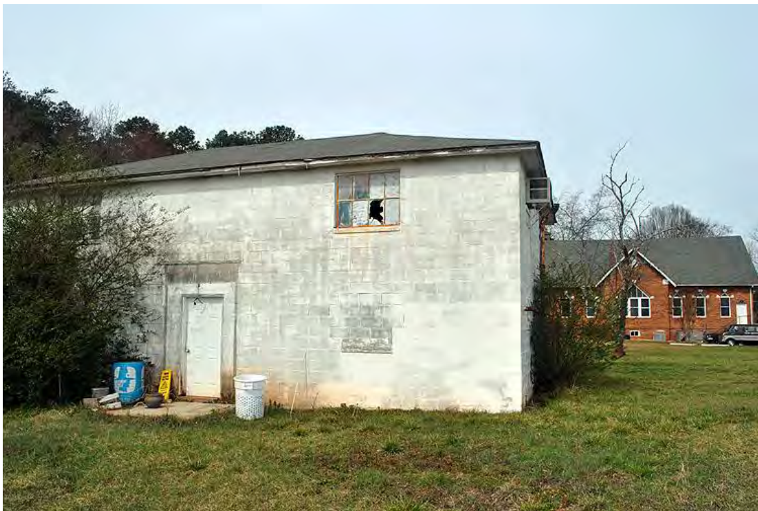
Hiram Masonic Lodge No. 22, South (Rear) Elevation, Looking North
