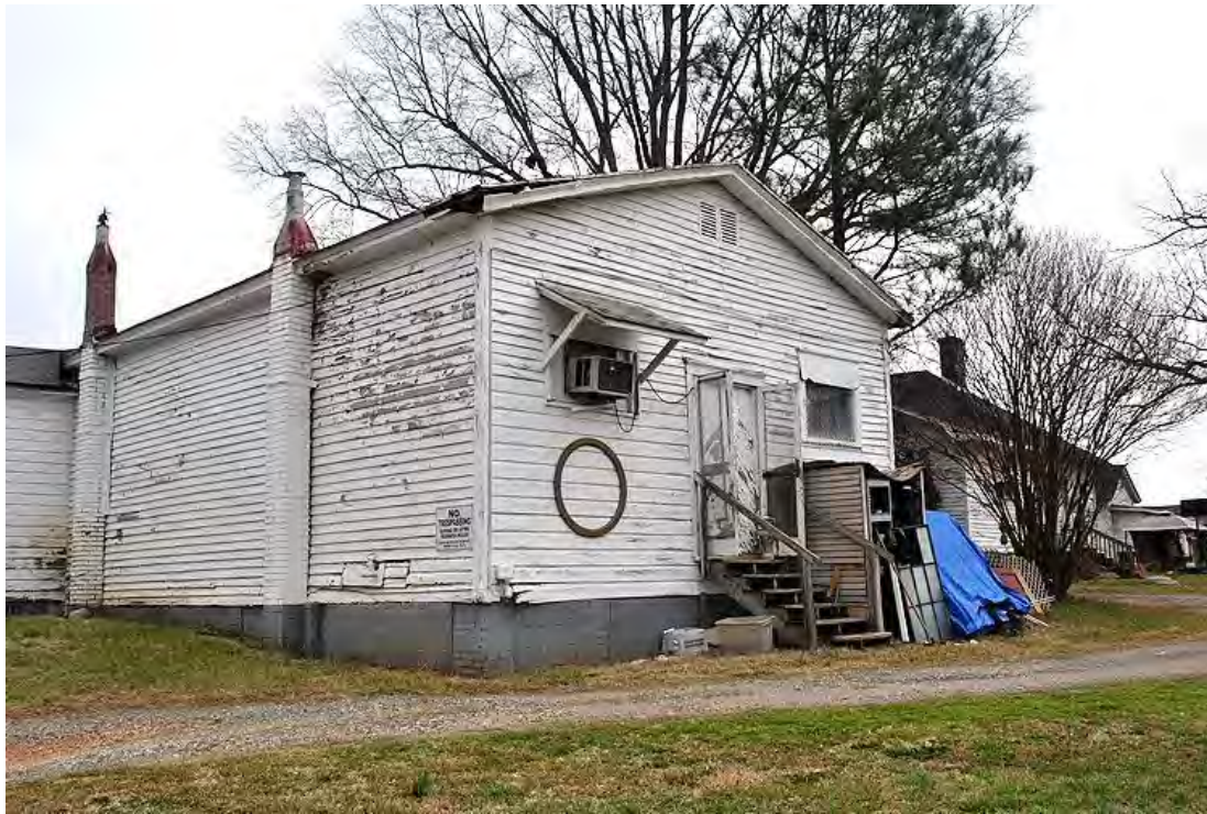
Nipper House and Store, Store, Rear (South) Elevation, Looking North.
