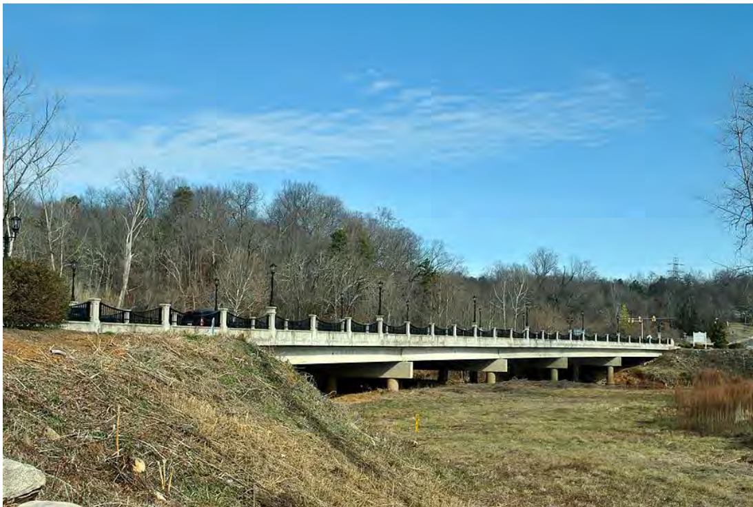
McAdenville Historic District (No. 3), New Bride over South Fork of the Catawba River.
