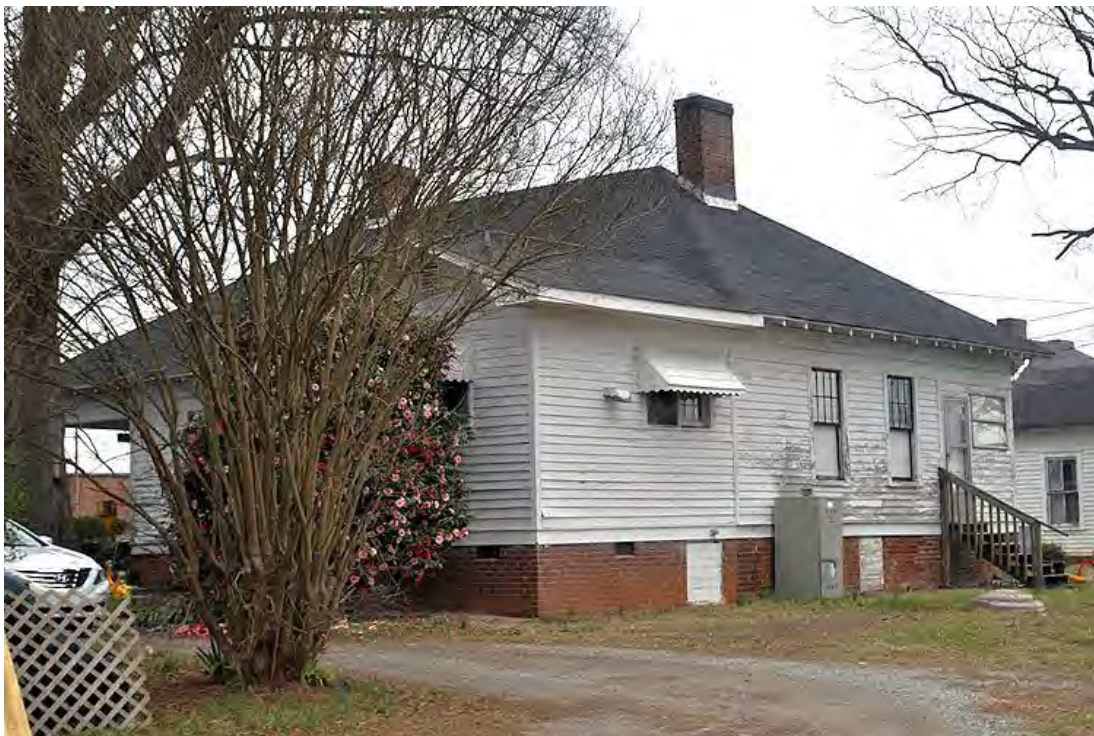
Nipper House and Store, House, 1950s Addition and Rear (South) Elevation, Looking North.
