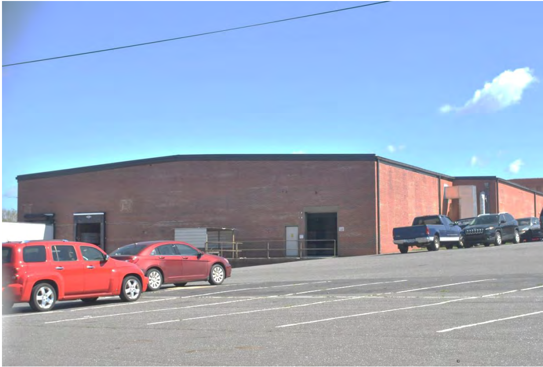
Groves Mills, Dye House/Finishing Plant, West Wing, Looking East from Apple Street.
