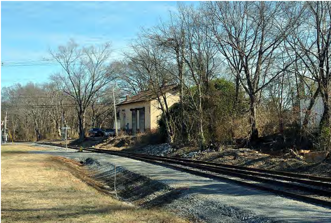
Piedmont and Northern Railway Linear Historic District, Piedmont and Northern Railway and Electrical Substation at North Modena Road (Within the APE), Gastonia, Looking East.
