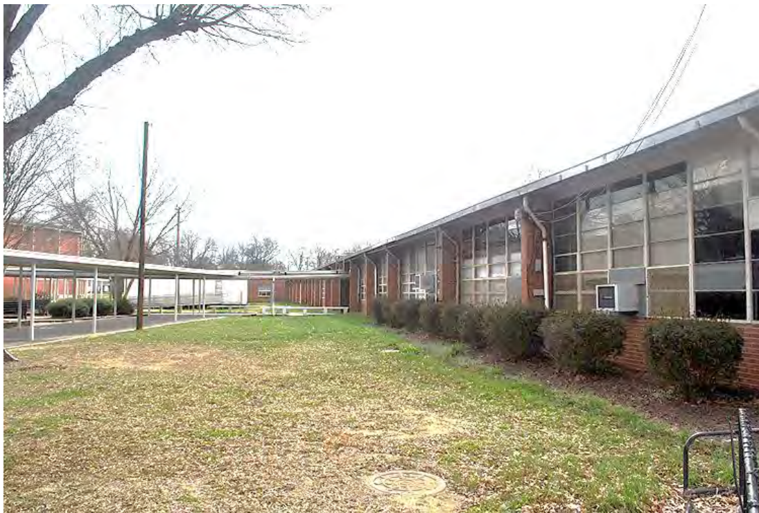
Holbrook High School, West Classroom Building, Side (East) Elevation, Looking South.
