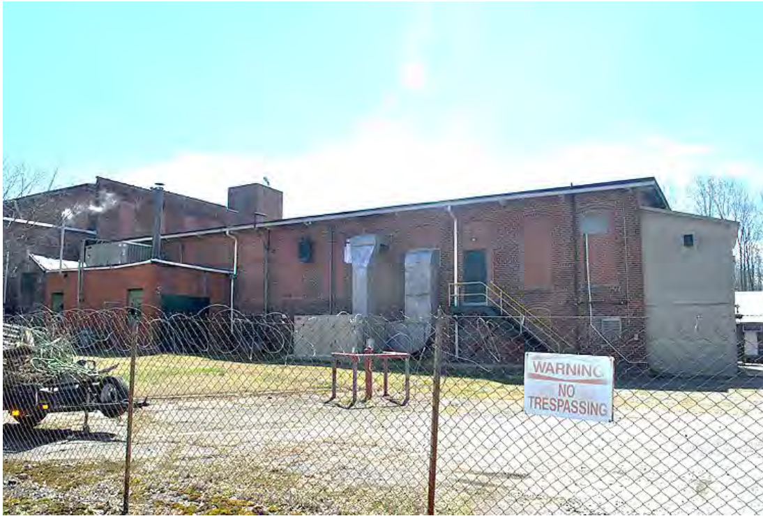
Modena Cotton Mills, Mill No. 1, 1896 Rear Wing, Side (North) Elevation, Looking South.
