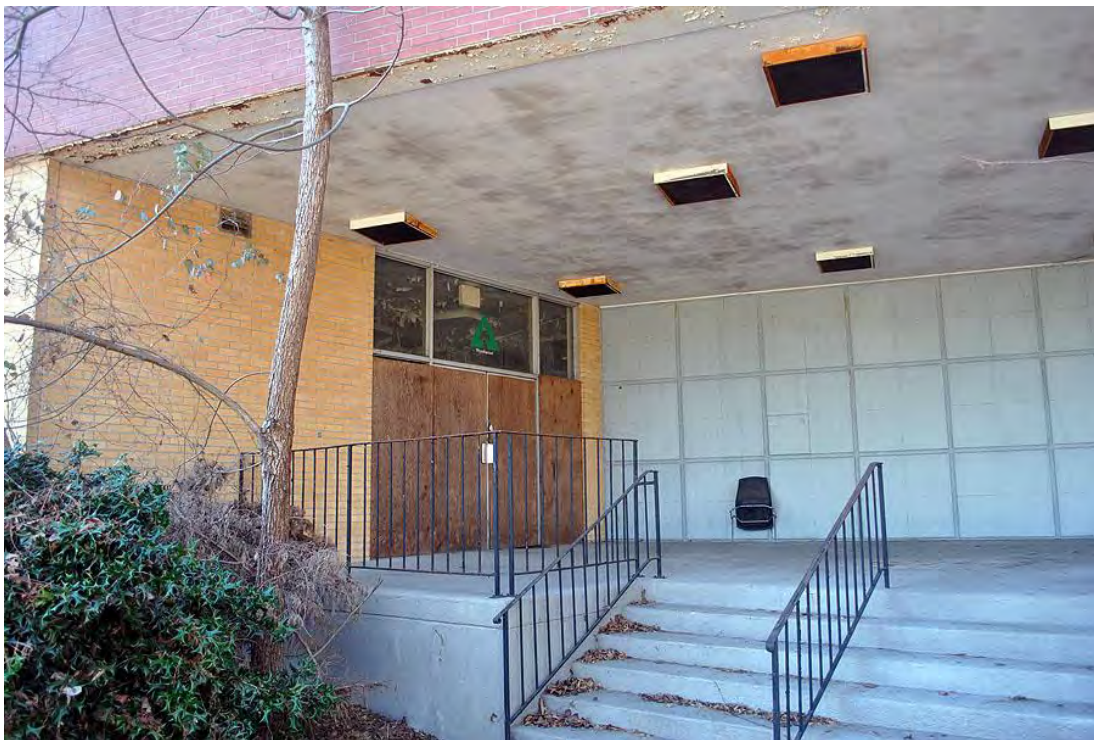
Hinde and Dauch Paper Company Factory, North Bay Porch and Entrance.
