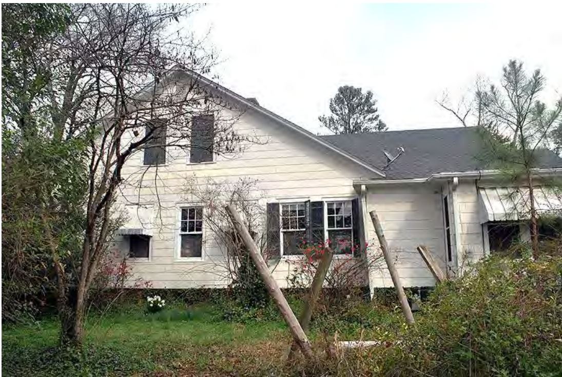
Paul P. and Virginia R. Murphy House, Side (South) Elevation, Looking North.
