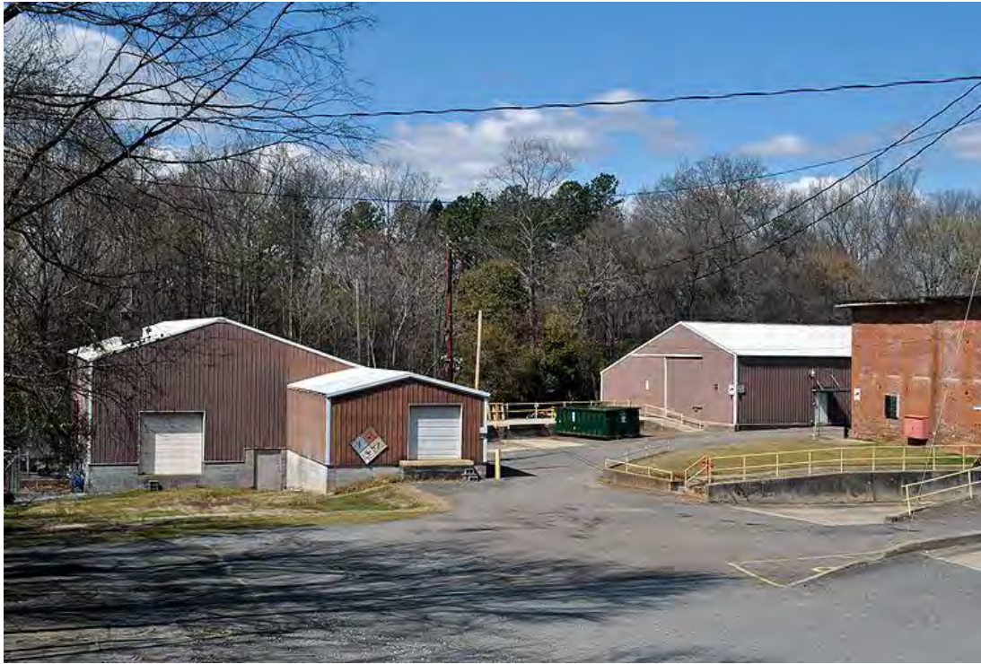
Modena Cotton Mills, Modern Storage Buildings, Looking West.
