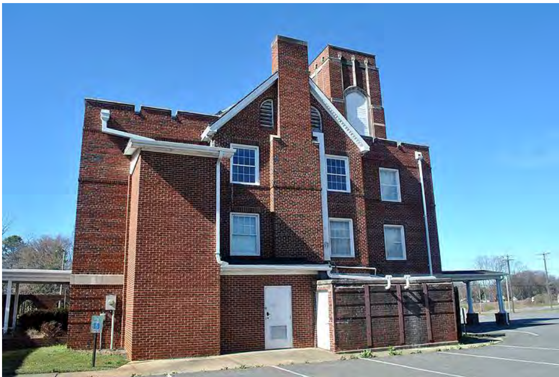
Faith United Methodist Church, East (Rear) Elevation, Looking West.
