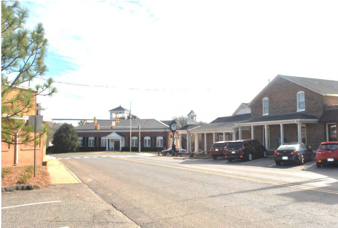
Pharr Corporate Offices, 100 Main Street, McAdenville (in Background), Looking East.
