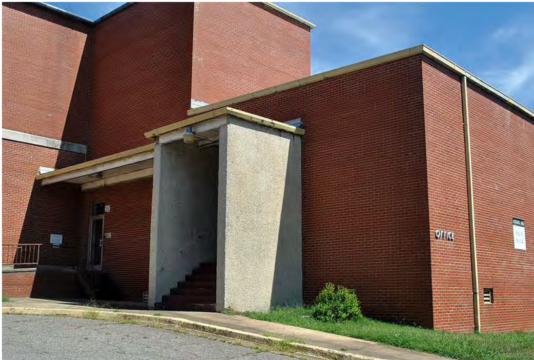
Flint Manufacturing Company, Mill No. 2, Office (circa 1950), Looking North.
