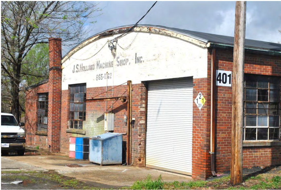
Gastonia Textile Machinery Company, Rear (South) Elevation, Looking North.
