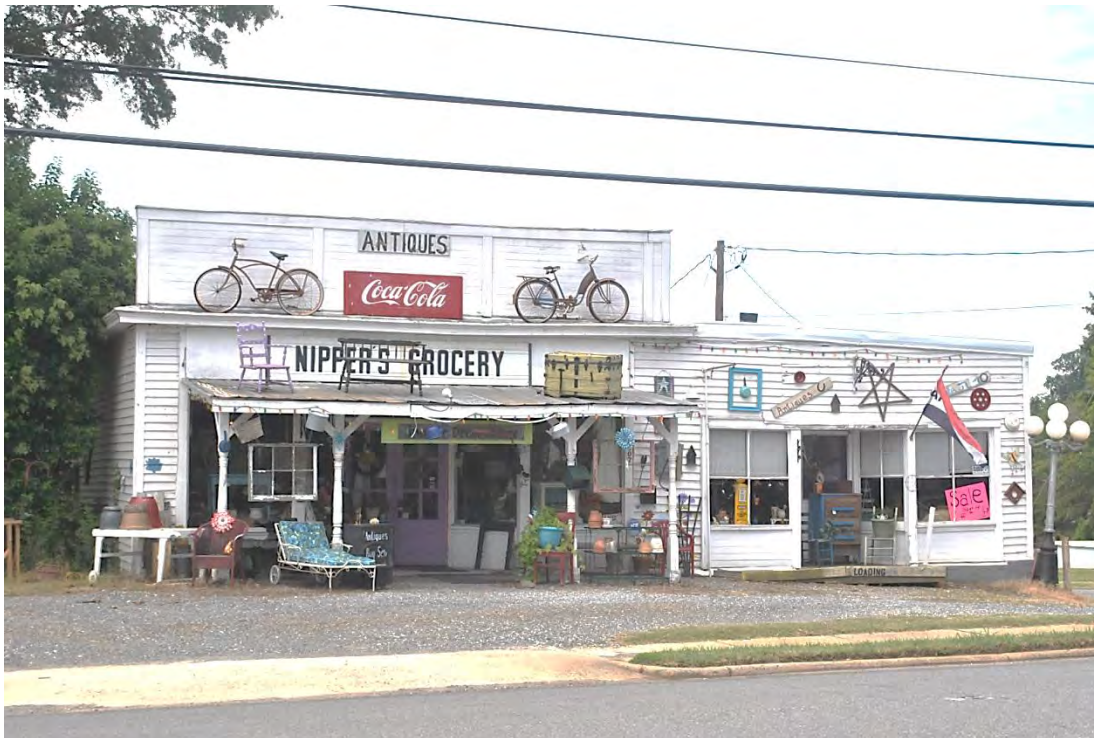
Nipper House and Store, Store, Façade, Looking South.
