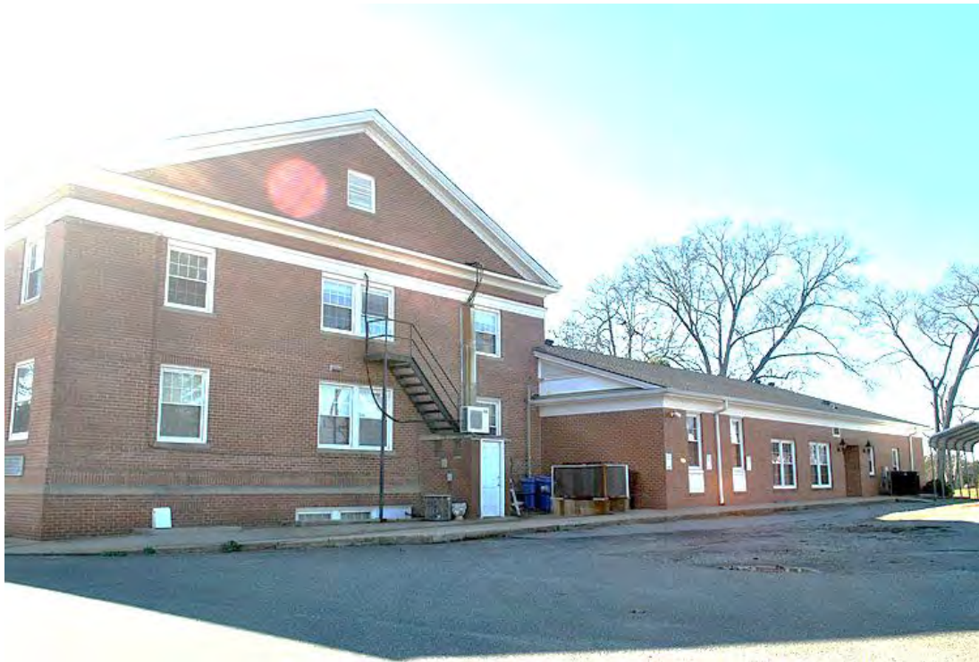
First Baptist Church of Lowell, Rear (North) Elevation and Fellowship Hall, Looking Southwest.
