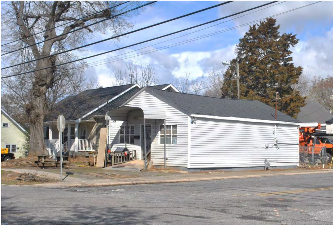
West Second Street Grocery (in Loray Mill Historic District), 700 West Second Avenue, Gastonia Looking Northwest.
