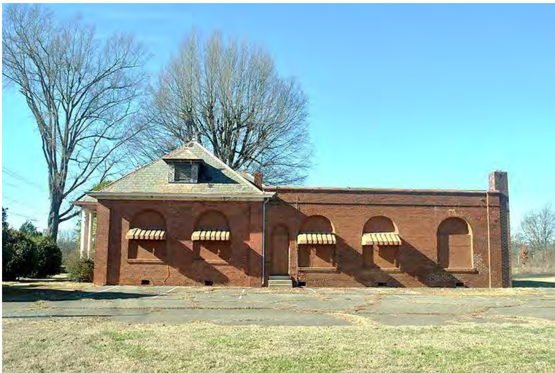
Lowell Cotton Mills, Mill Office, Side (East) Elevation, Looking West.
