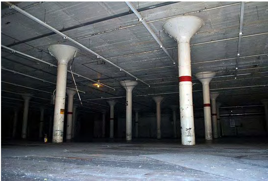
Flint Manufacturing Company, Mill No. 2, Interior, First Floor, Main Manufacturing Room.
