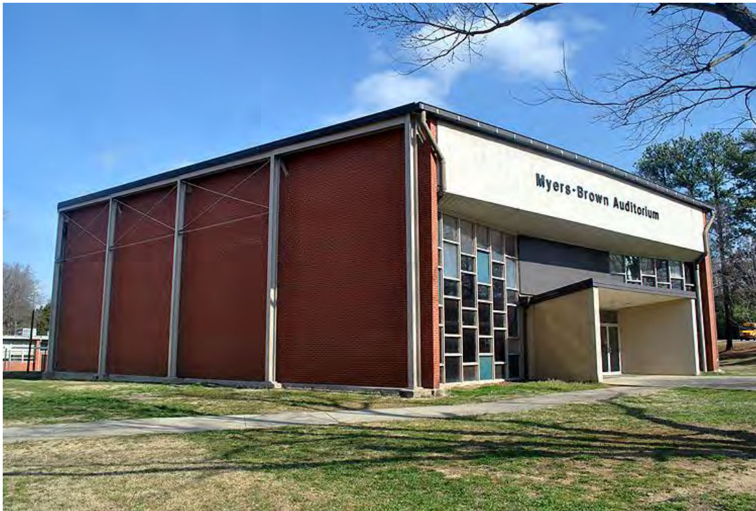
Holbrook High School, Auditorium, Looking Northeast.
