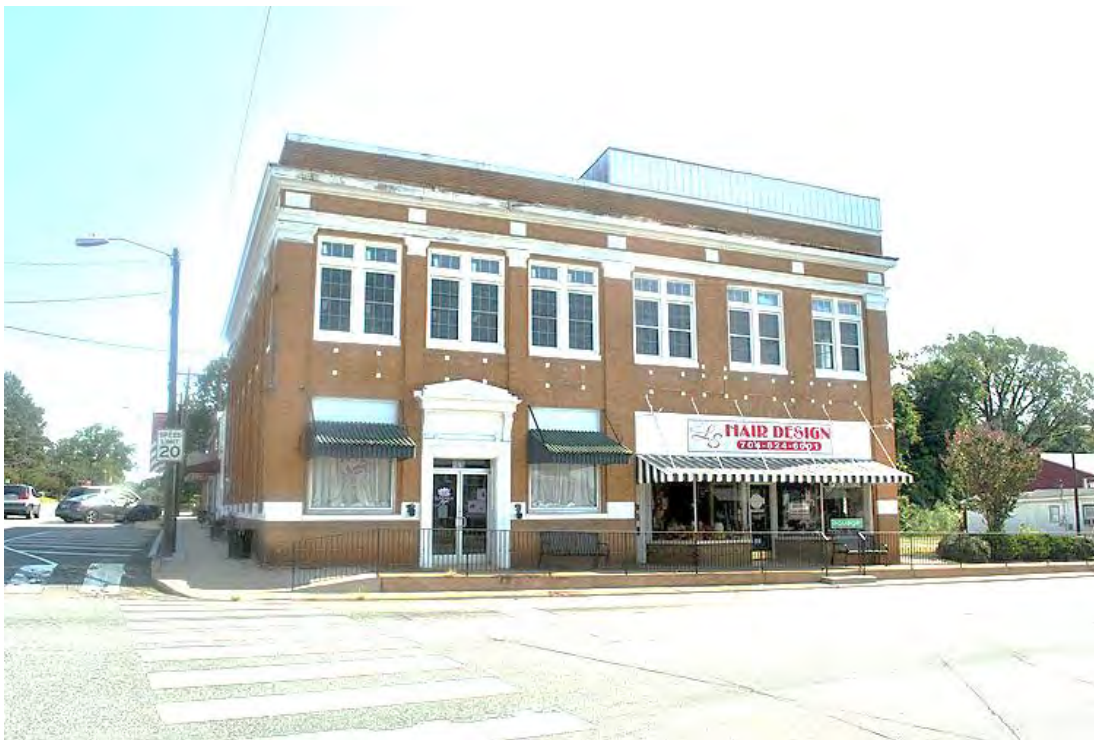
Lowell Historic District, Bank of Lowell, 101-105 East First Street, Looking North.
