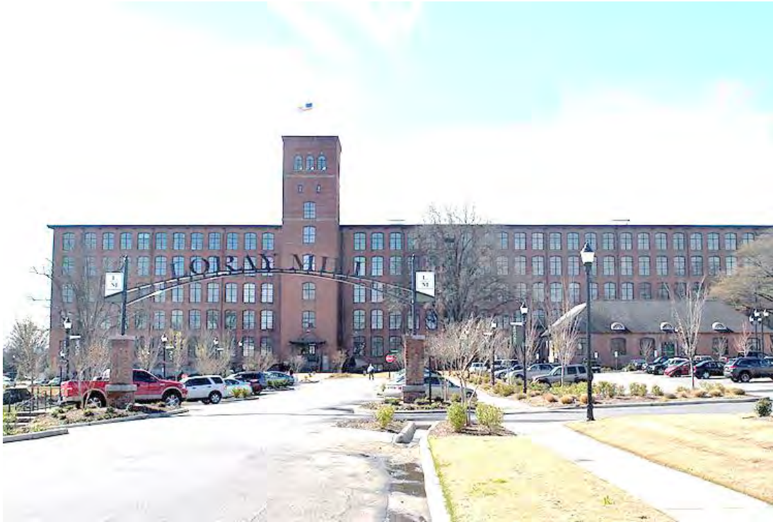
Loray Mill, 300 South Firestone Street, Gastonia, Mill Office on Right, Looking South.
