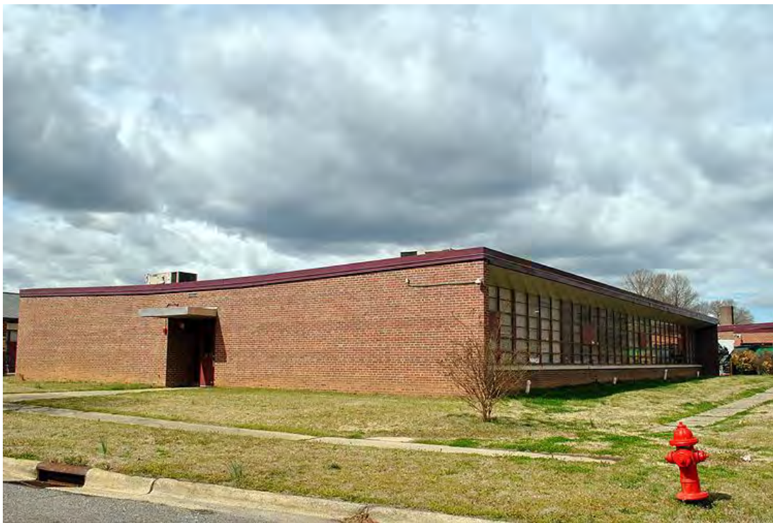
Victory Mills Grade School, 1601 Madison Street, Gastonia, Looking West.
