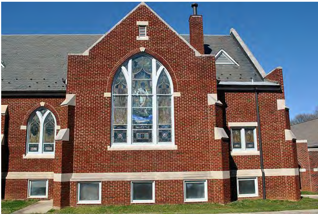
Lutheran Chapel and Cemetery, Side (South) Elevation and South Transept, Looking North.
