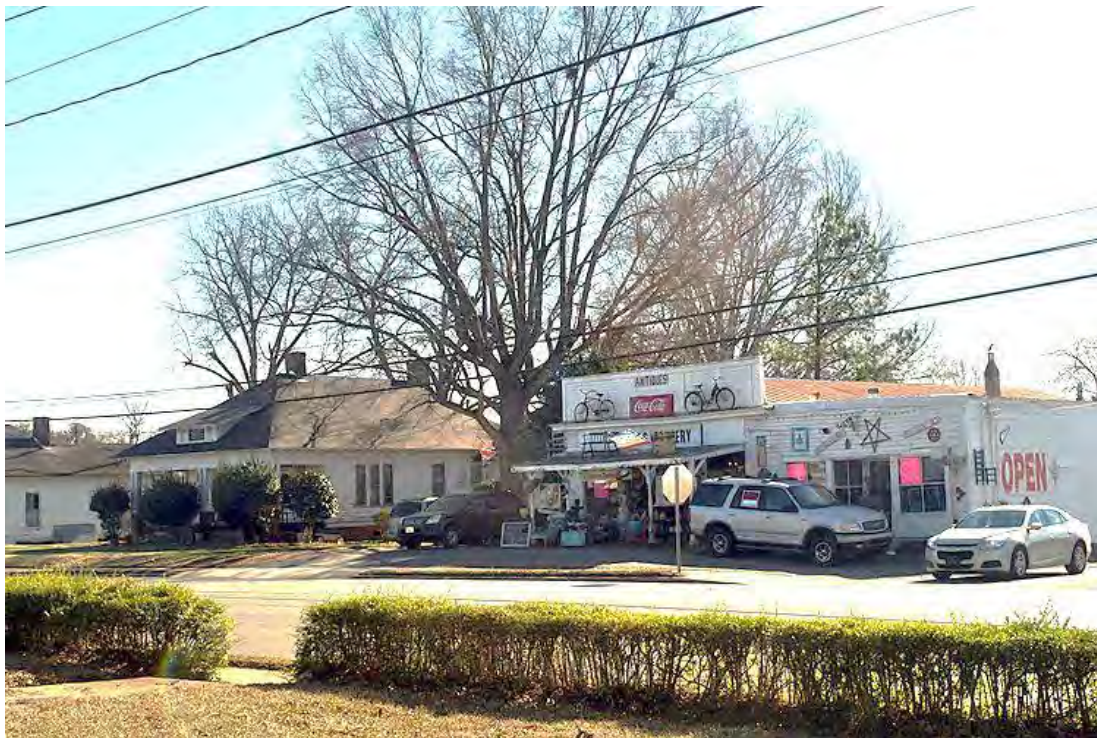
Nipper House and Store, Overall View, Looking Southeast.
