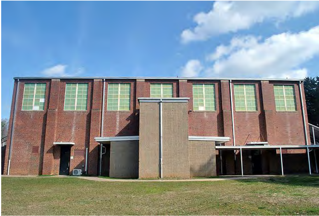
Holbrook High School, Gymnasium, South Elevation, and Entrance Bay Addition, Looking North.
