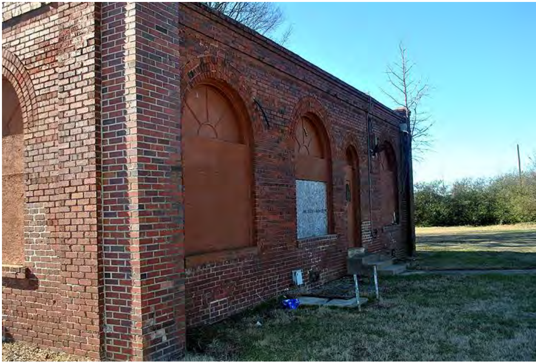
Lowell Cotton Mills, Mill Office, Rear (North) Elevation, Looking West.
