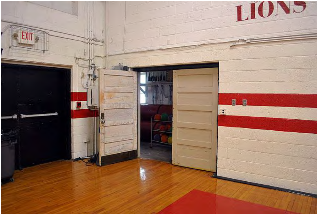
Holbrook High School, Gymnasium, Doorway to Equipment Room.
