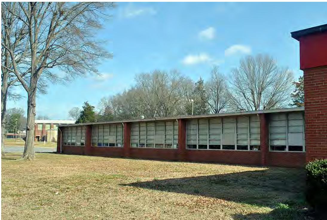
Holbrook High School, West Classroom Building, 1954 Side (West) Elevation, Looking North.
