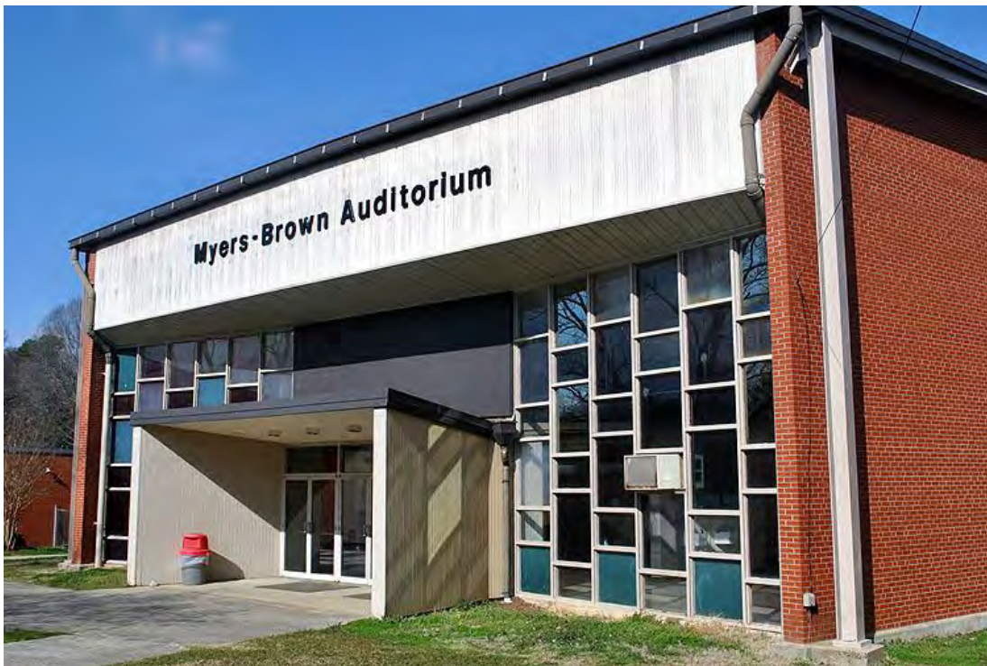
Holbrook High School, Auditorium, Façade (South Elevation), Looking Northwest.
