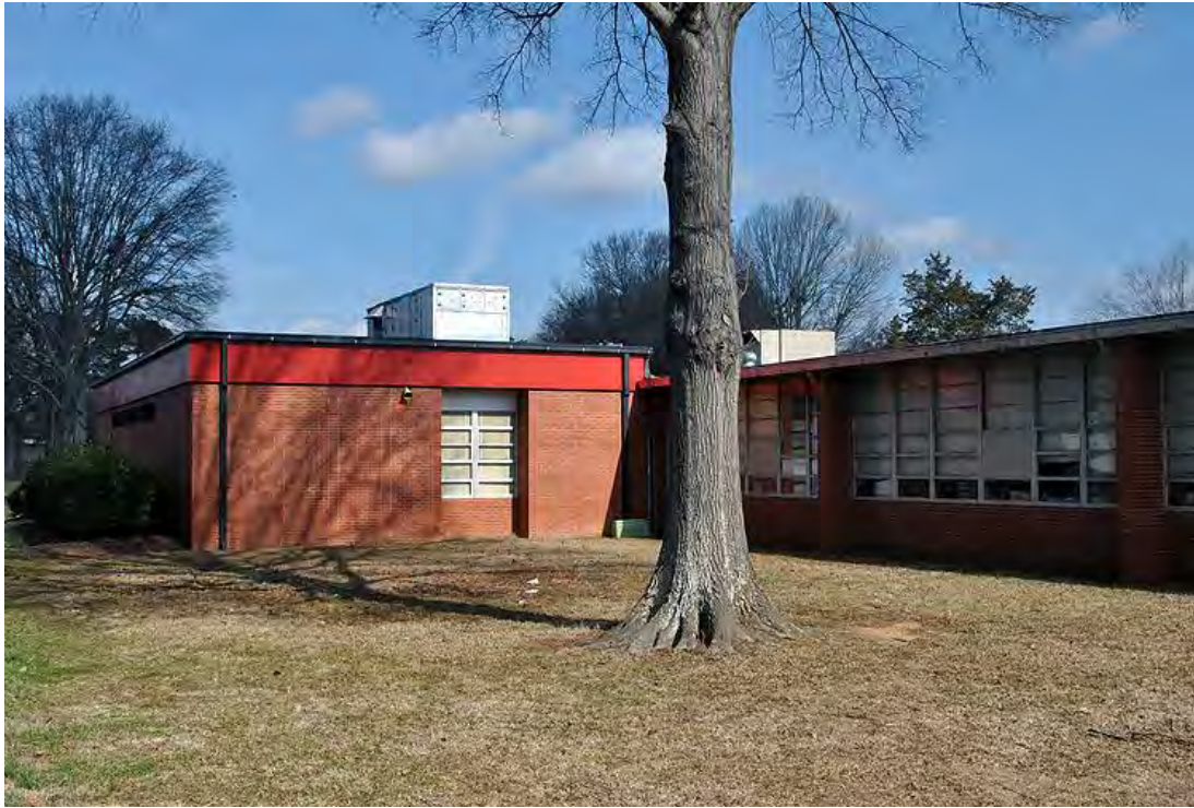
Holbrook High School, 1975 Addition to West Classroom Building Side (West) Elevation, Looking North.
