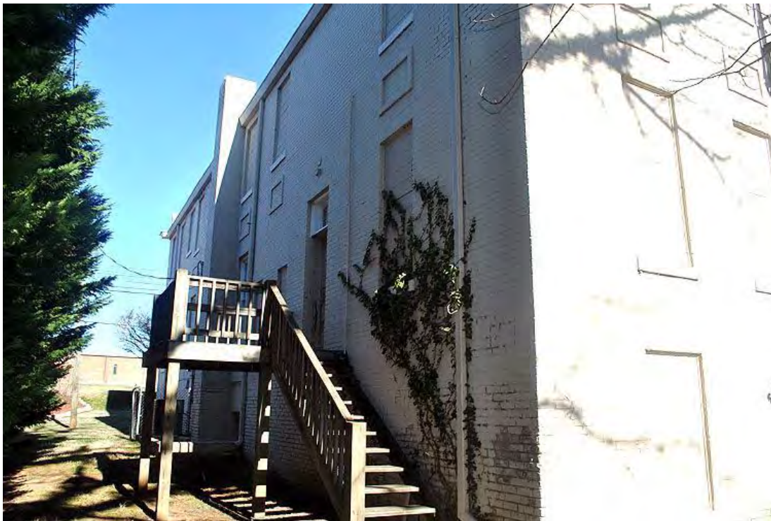
Lowell Teacherage, Rear (West) and Side (South) Elevations, Looking North.
