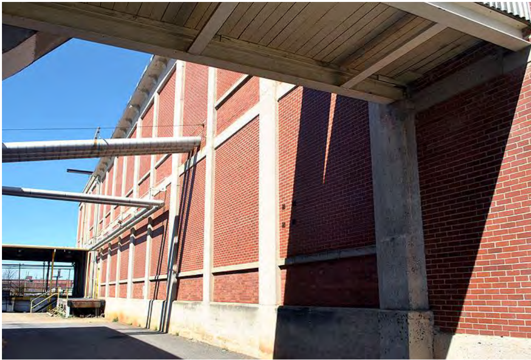
Flint Manufacturing Company, Mill No. 2, Side (West) Elevation, Looking North.
