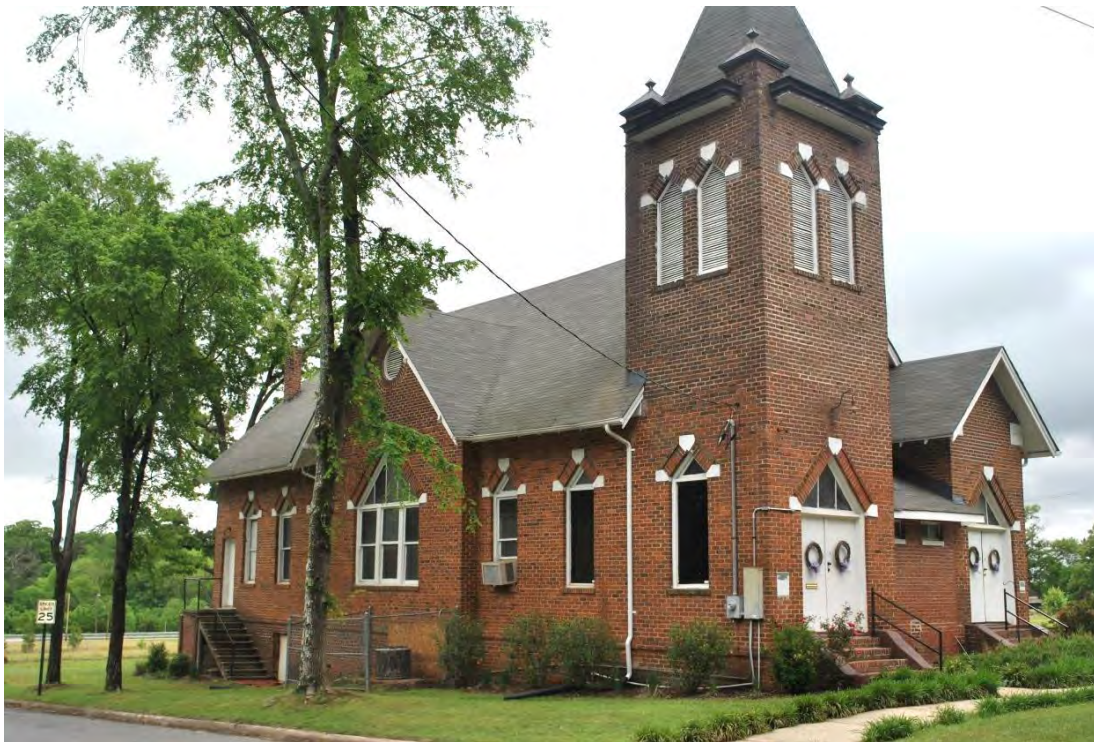
Wrights Chapel A.M.E. Zion Church, Front (West) and Side (North) Elevations, Looking Southeast.
