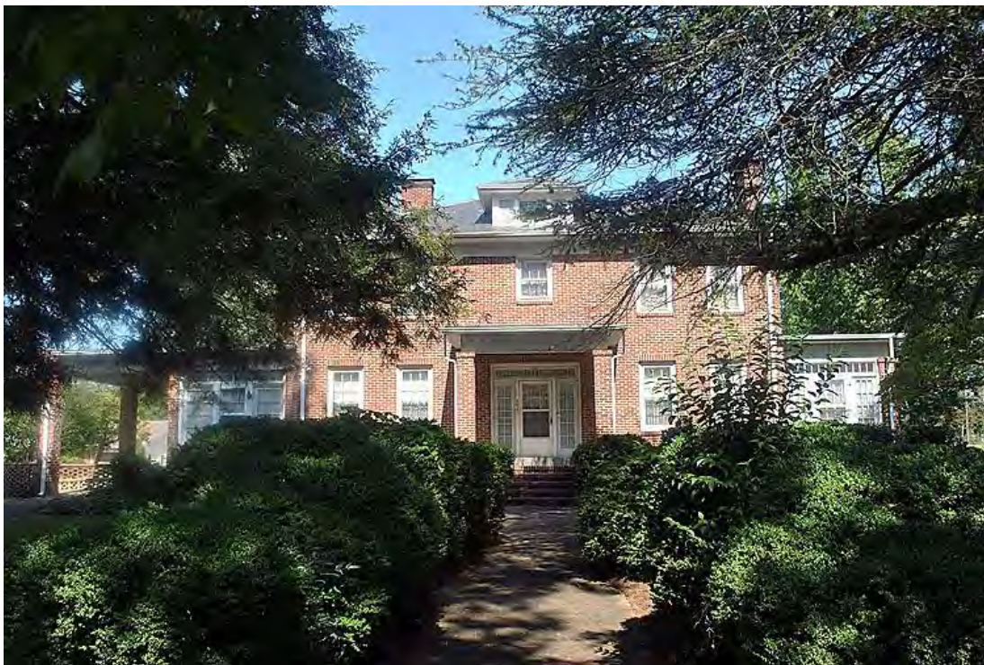
Lowell Historic District, Dr. James W. and Jennie Reid House, 201 Mill Street, Looking West.
