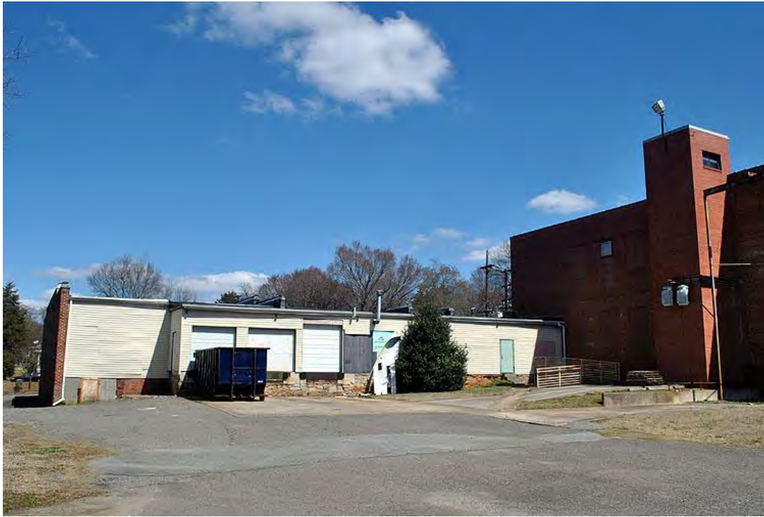
Modena Cotton Mills, Mill No. 2, Cotton Warehouse (1905), South Elevation, Looking North.
