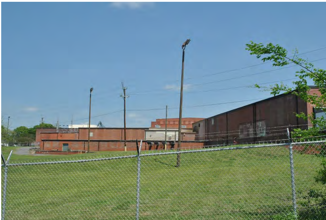
Groves Mills, Dye House/Finishing Plant, West Elevations, Looking East from Apple Street.
