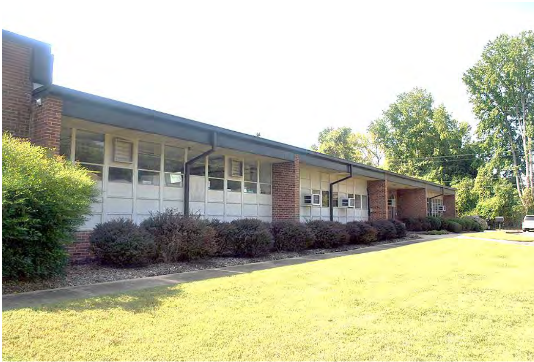
Dora R. Humphrey Elementary School, Façade (North Elevation), Looking West.
