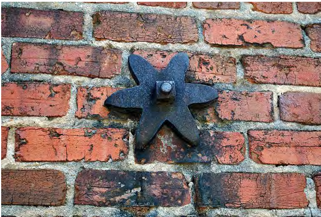
Modena Cotton Mills, Mill No. 2, Cotton Warehouse (1905), West Elevation, Tie-Rod Plate.
