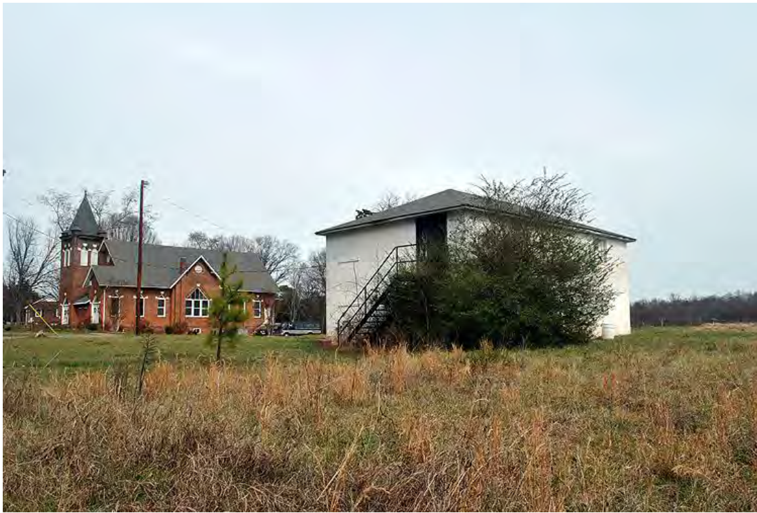
Hiram Masonic Lodge No. 22, Rear (South) and Side (West) Elevations, Looking North towards Wrights Chapel A.M.E. Zion Church.
