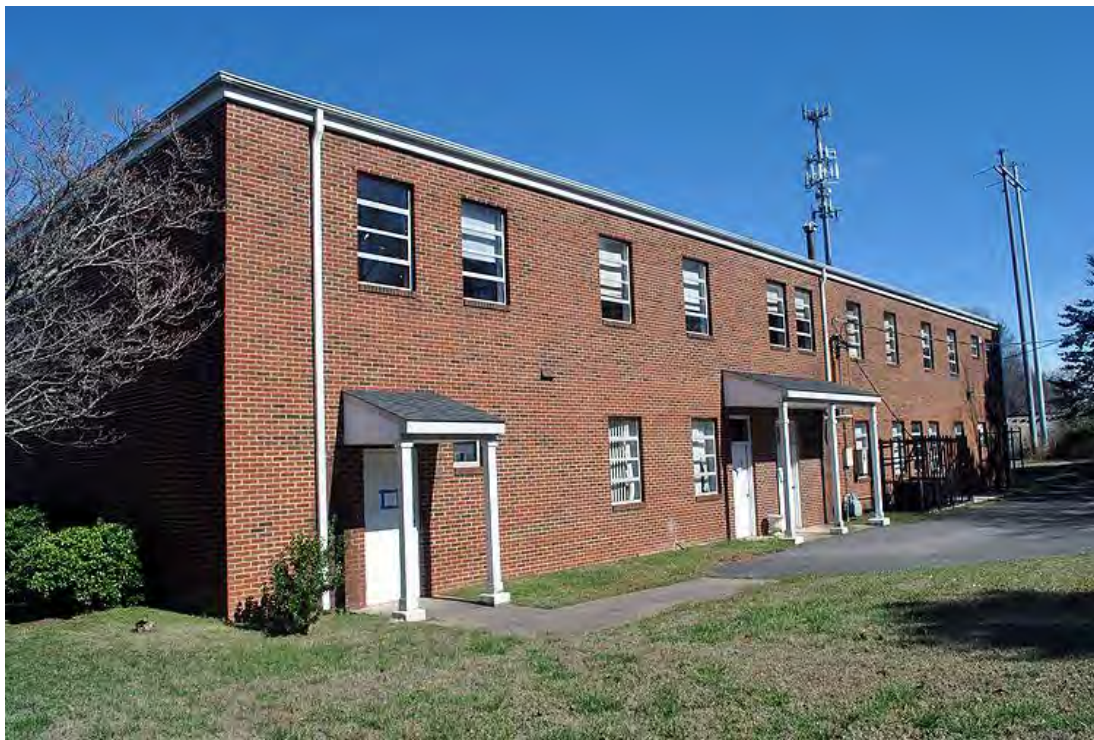
Faith United Methodist Church, Education Building, (Side) South Elevation, Looking Northeast.
