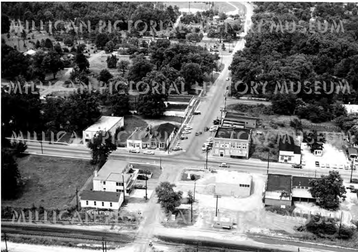
AERIAL VIEW MAIN STREET, LOWELL, NORTH CAROLINA
