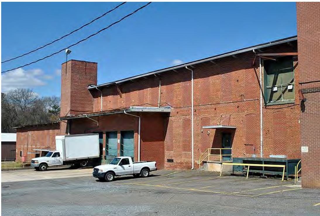
Modena Cotton Mills, Mill No. 1, 1894 Side (South) Elevation, Looking Northwest.
