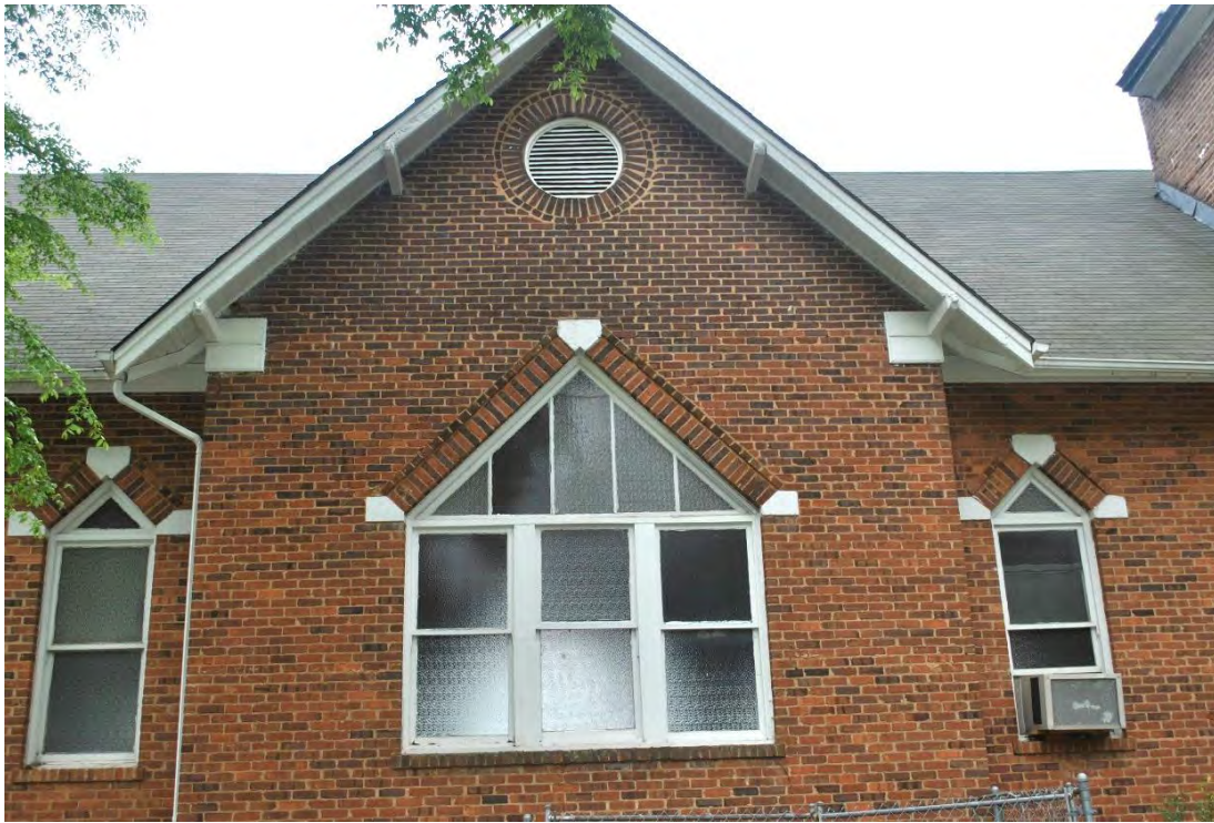
Wrights Chapel A.M.E. Zion Church, Side (North) Elevation, Looking South.
