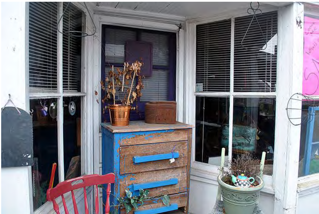
Nipper House and Store, Side Extension, Entrance Detail.
