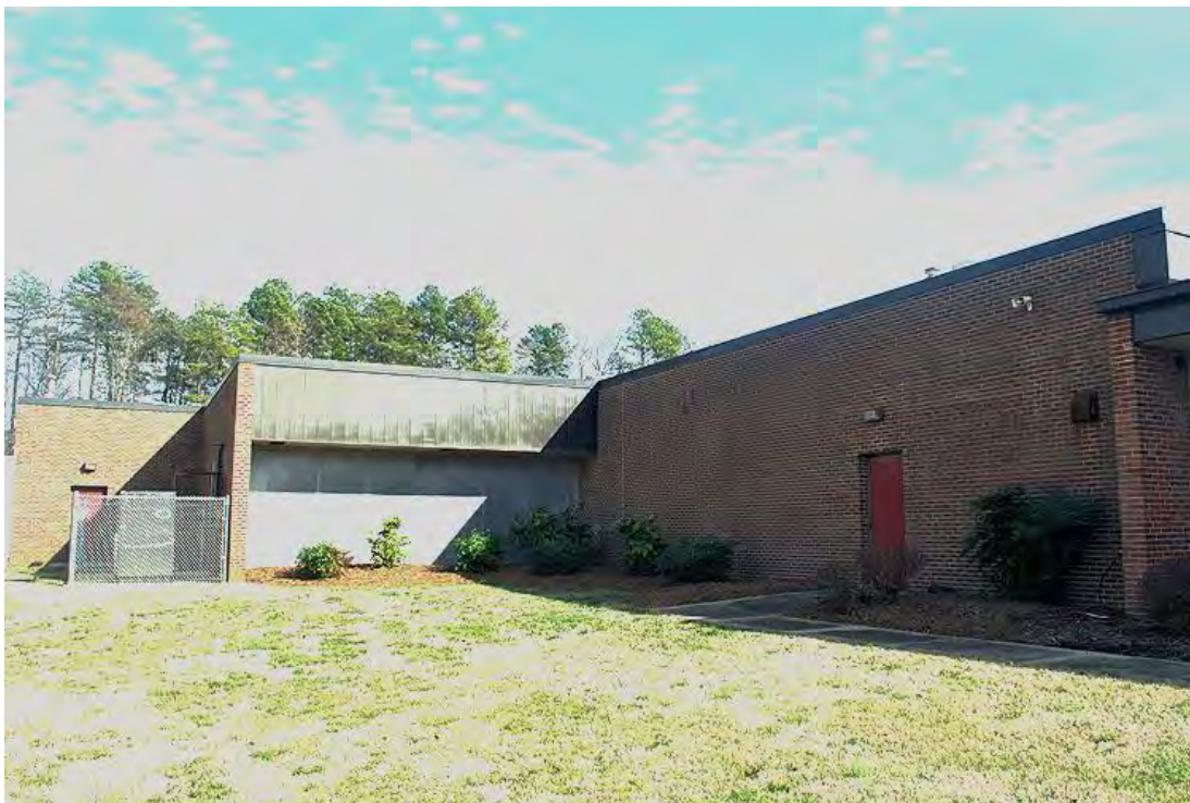
Dora R. Humphrey Elementary School, 1988 Addition, Looking Southeast.
