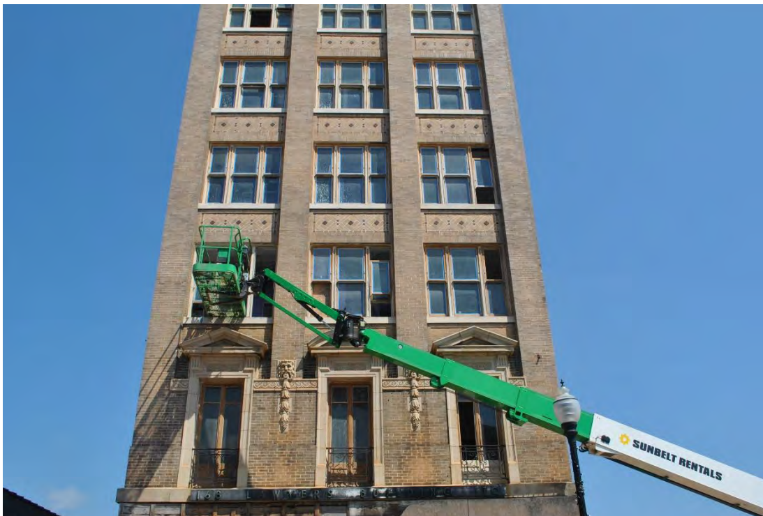
First National Bank, 168-170 West Main Avenue, Gastonia, Looking North.
