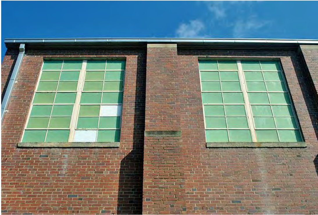
Holbrook High School, Gymnasium, South Elevation, Window Bays.
