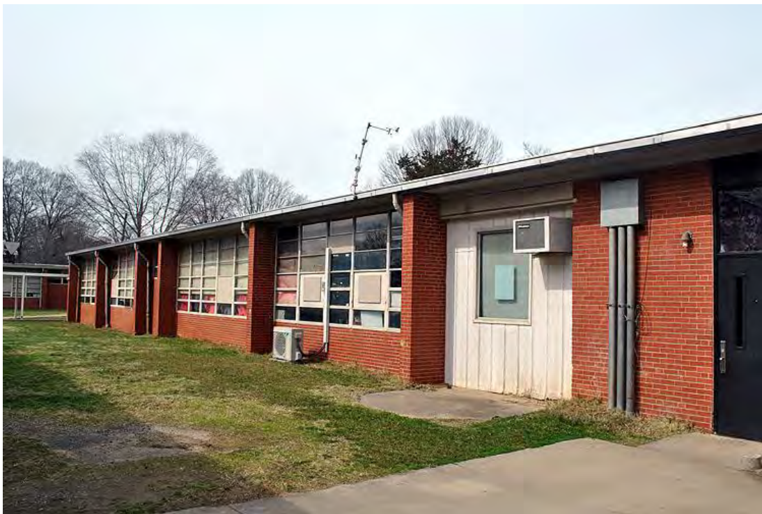
Holbrook High School, East Classroom Building, South Elevation, Looking West.
