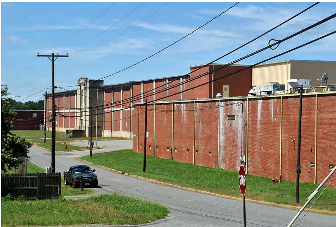
Flint Manufacturing Company, Mill No. 2, Overall View, Looking Northwest.
