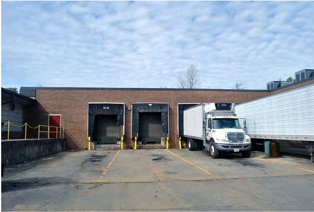
Dora R. Humphrey Elementary School, South (Rear) Elevation of 1988 Addition, Looking North.
