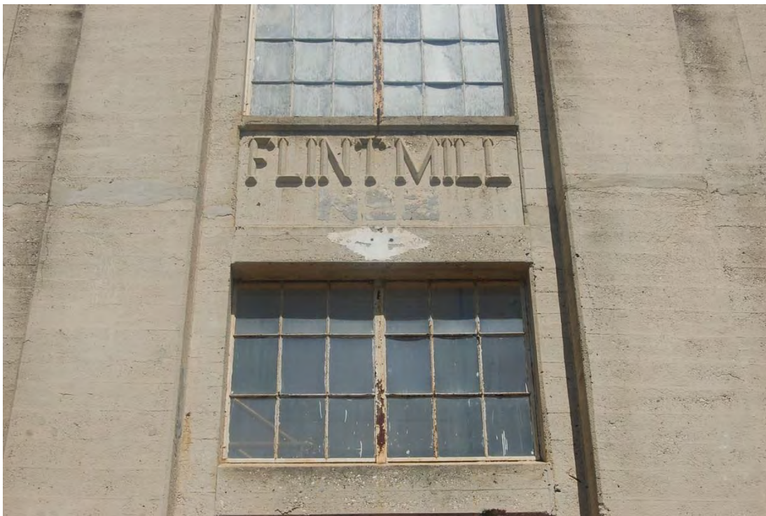
Flint Manufacturing Company, Mill No. 2, Main Entrance Detail.
