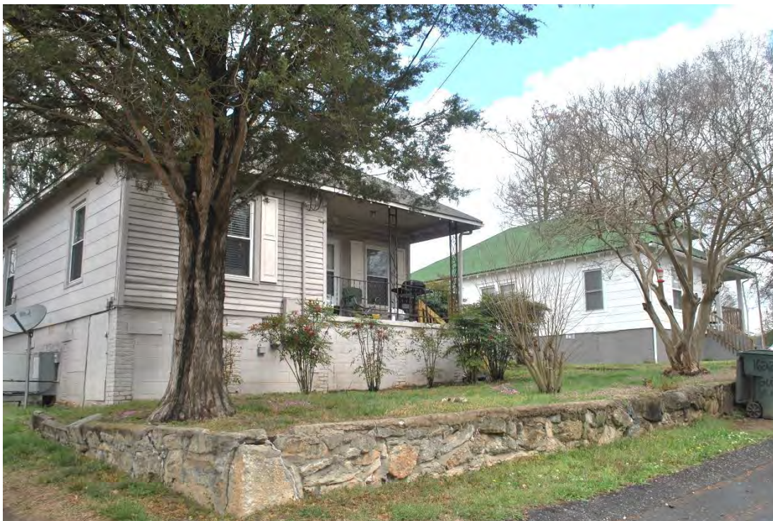
Groves Mill Village, 1600 Block of Gum Street, Looking Northeast.
