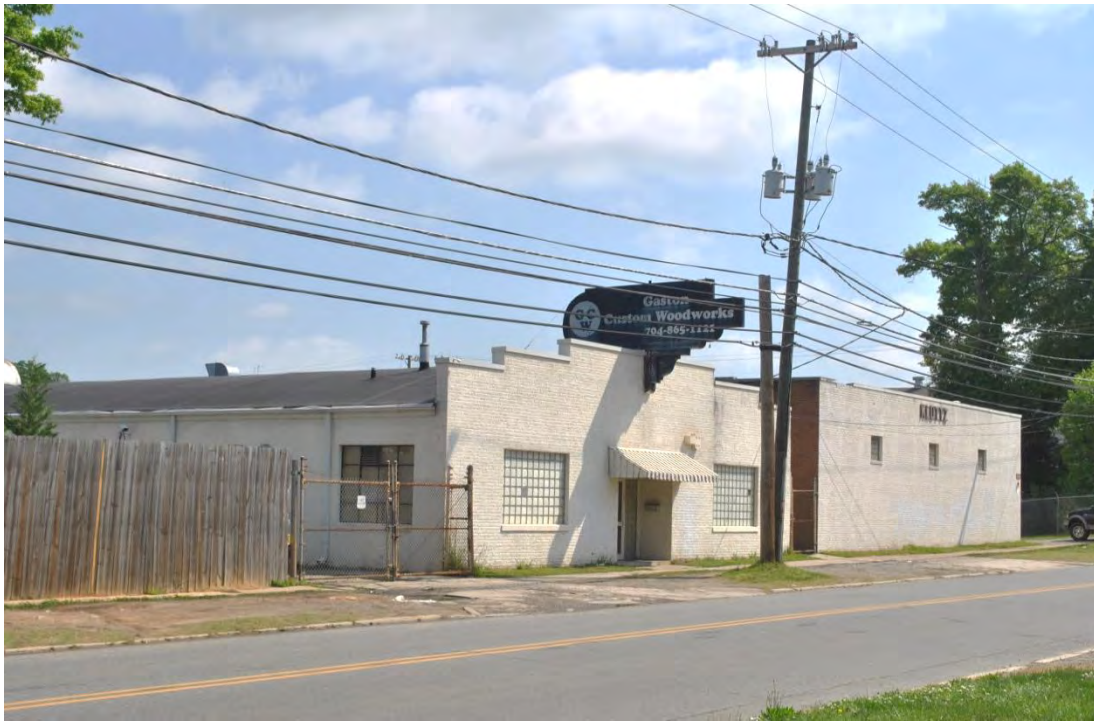
Todd-Long Picker Apron Corporation (Building on Left), 618 East Second Avenue, Gastonia, Looking Northeast.
