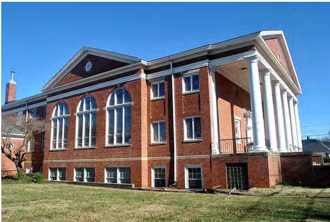
First Baptist Church of Lowell, Side (West) Elevation, Looking East.
