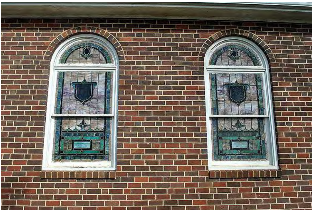
O'Conner's Grove A.M.E. Zion Church and Cemetery, South Elevation Windows.
