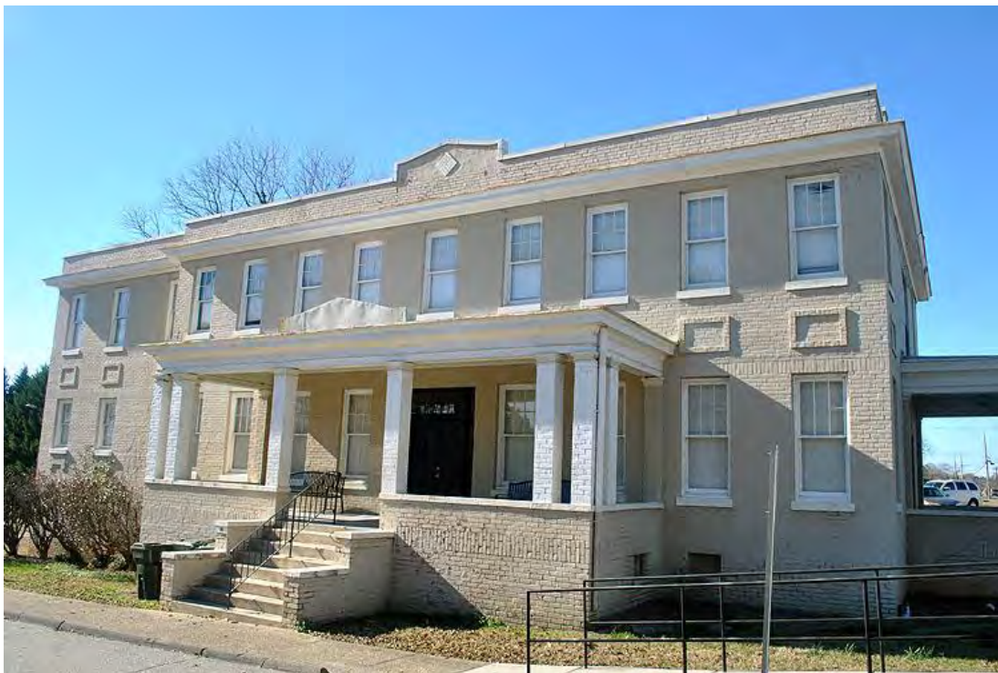
Lowell Teacherage, Façade (East Elevation), Looking West.
