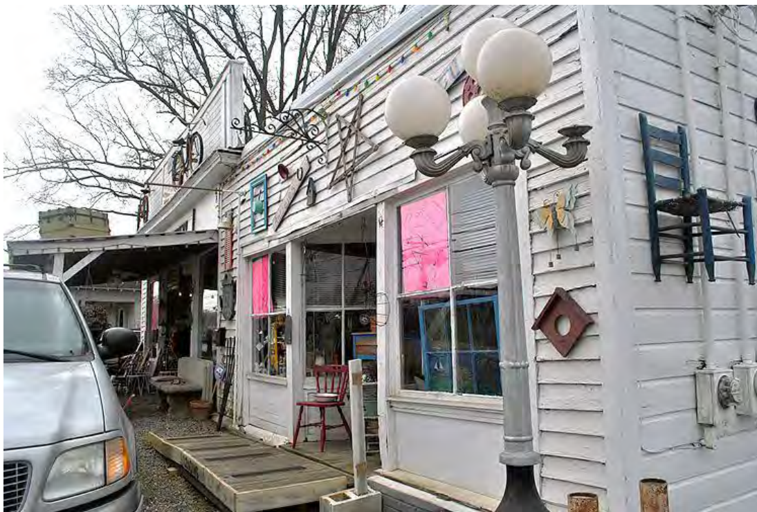
Nipper House and Store, Store, Façade, Looking Southeast.
