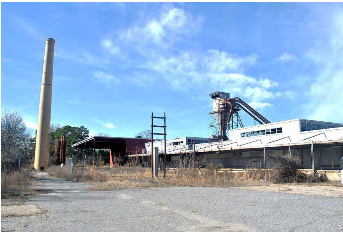
Hinde and Dauch Paper Company Factory, Production Building (Right), Shed, Water Tank, and Smoke Stack (Left), Looking North.
