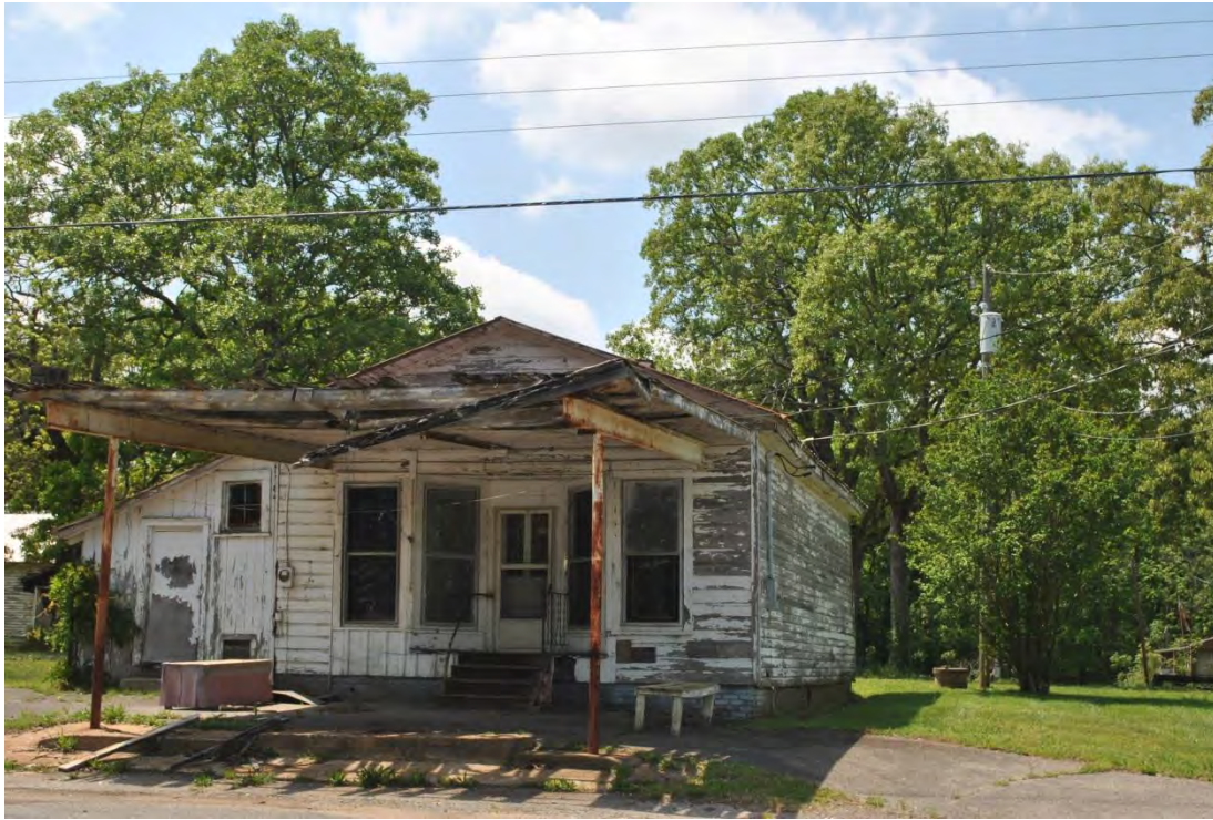
Farnsworth Store, 3101 Tryon Courthouse Road, Cherryville, Looking South.
