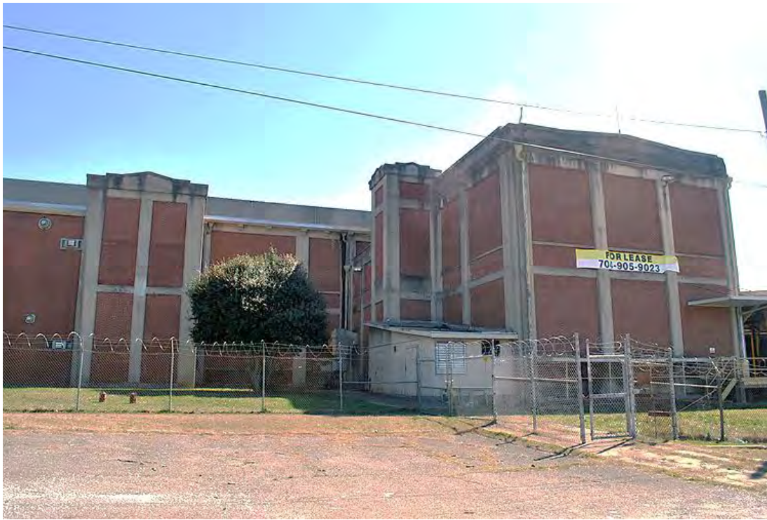
Flint Manufacturing Company, Mill No. 2, Rear (North) Elevation and Picker House Wing, Looking South.
