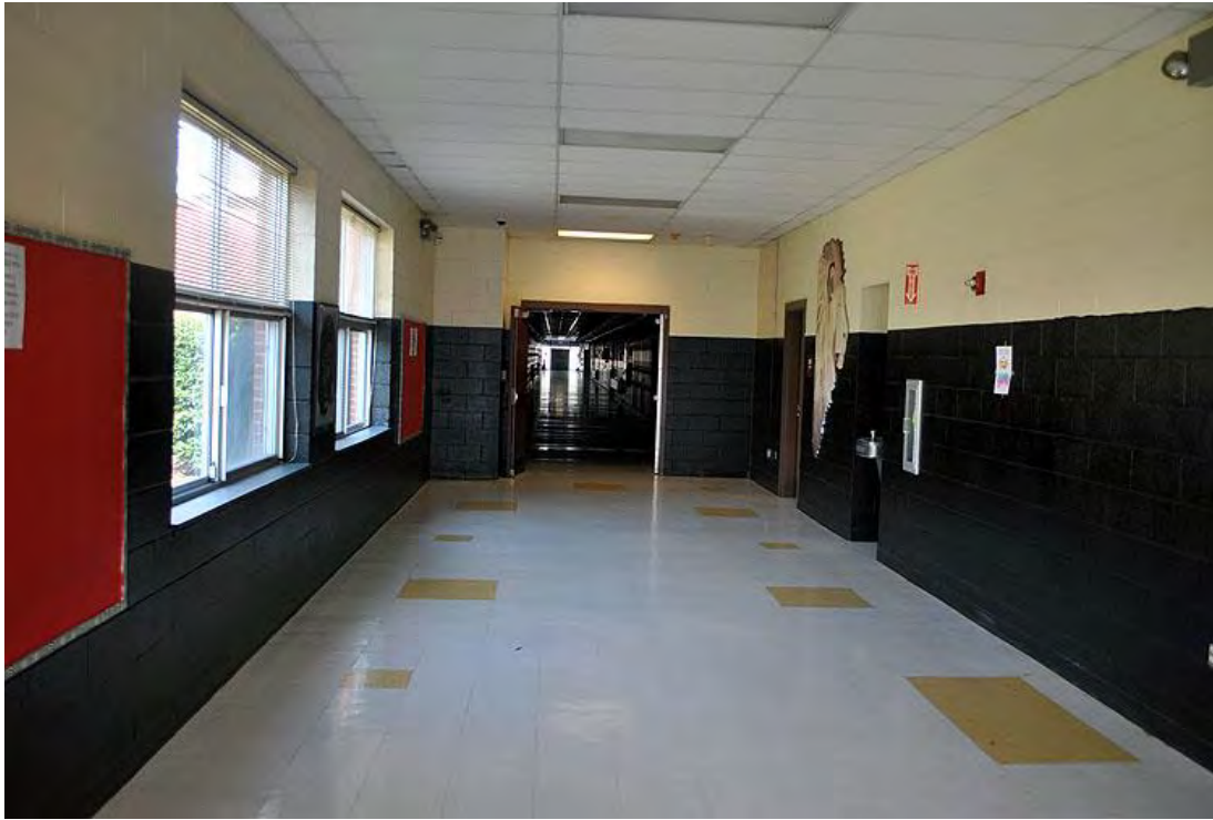
Holbrook High School, West Classroom Building, 2000 Middle School Façade Addition, Interior, Modern Entrance Corridor Leading to Original Entrance.
