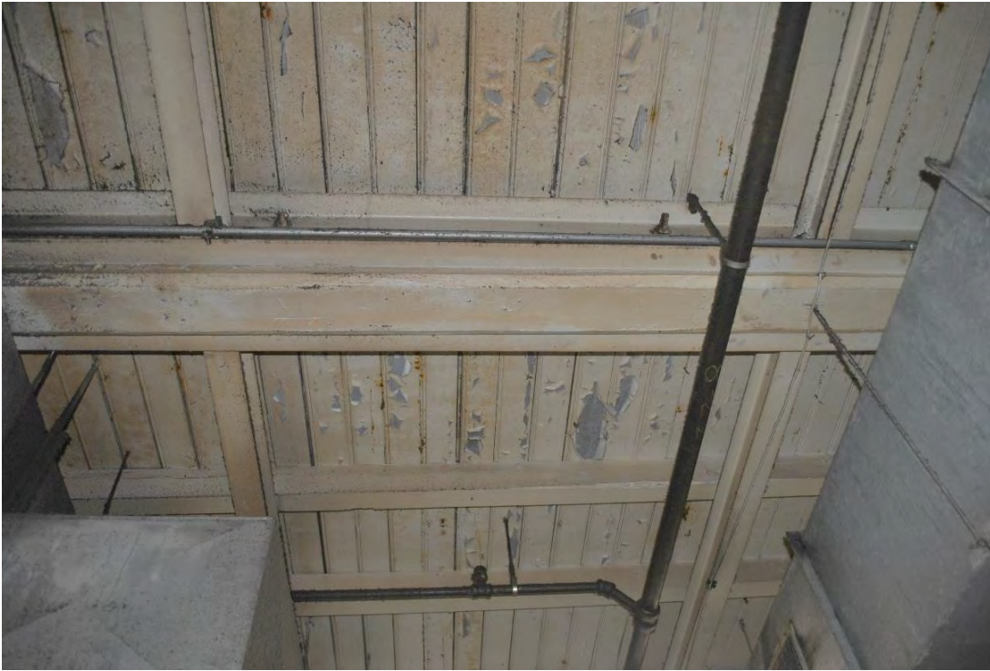
Modena Cotton Mills, Mill No. 1, Interior, Main Manufacturing Room (1894), Ceiling.
