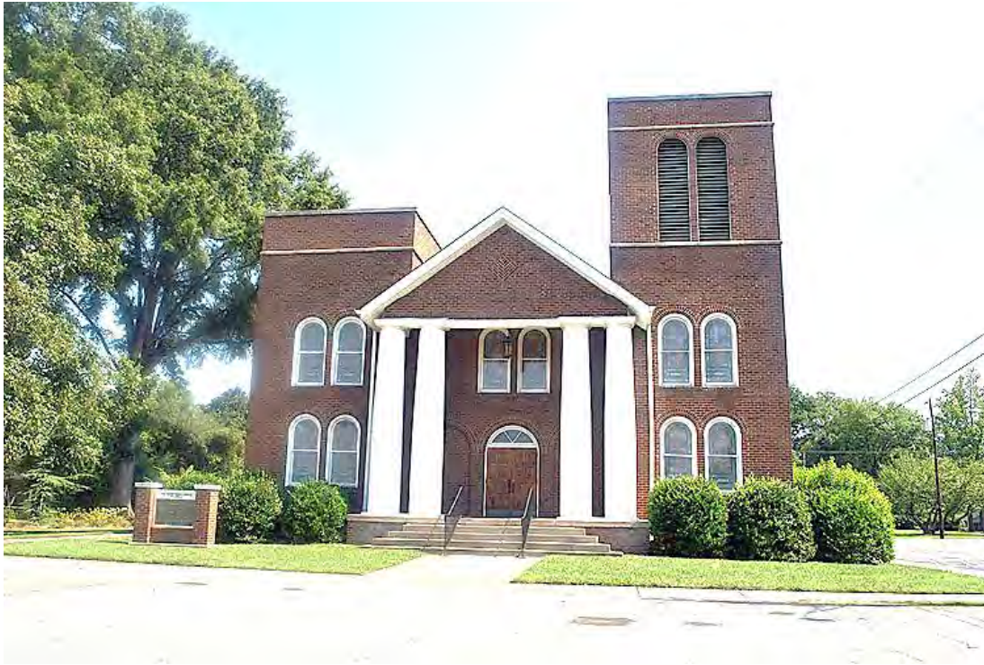
Lowell Historic District, Presbyterian Church of Lowell, 207 East First Street, Looking North
