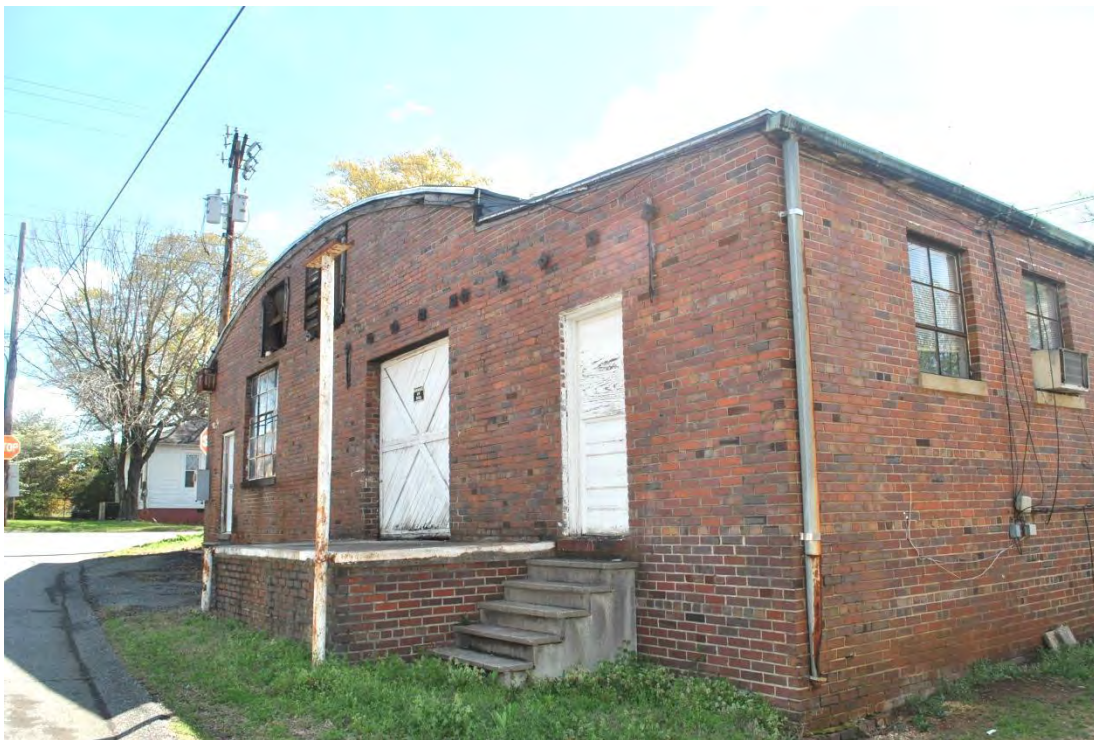
Gastonia Textile Machinery Company, Front (North) Elevation, Looking East.
