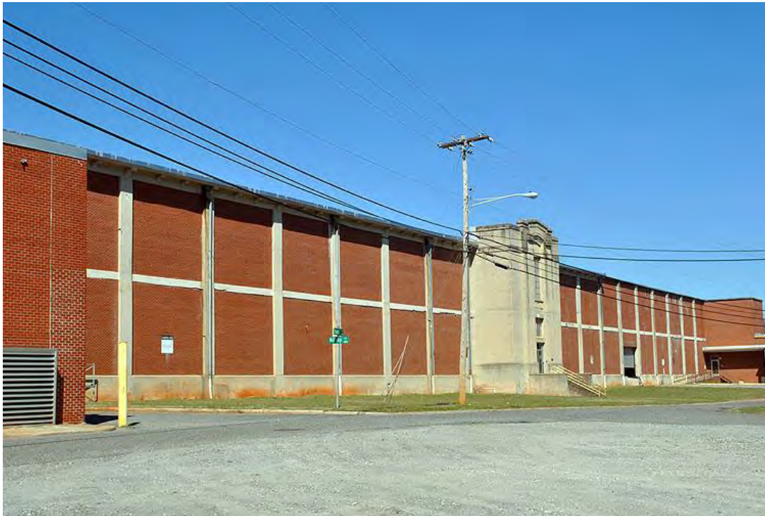
Flint Manufacturing Company, Mill No. 2, Façade (South Elevation), Looking Northeast.
