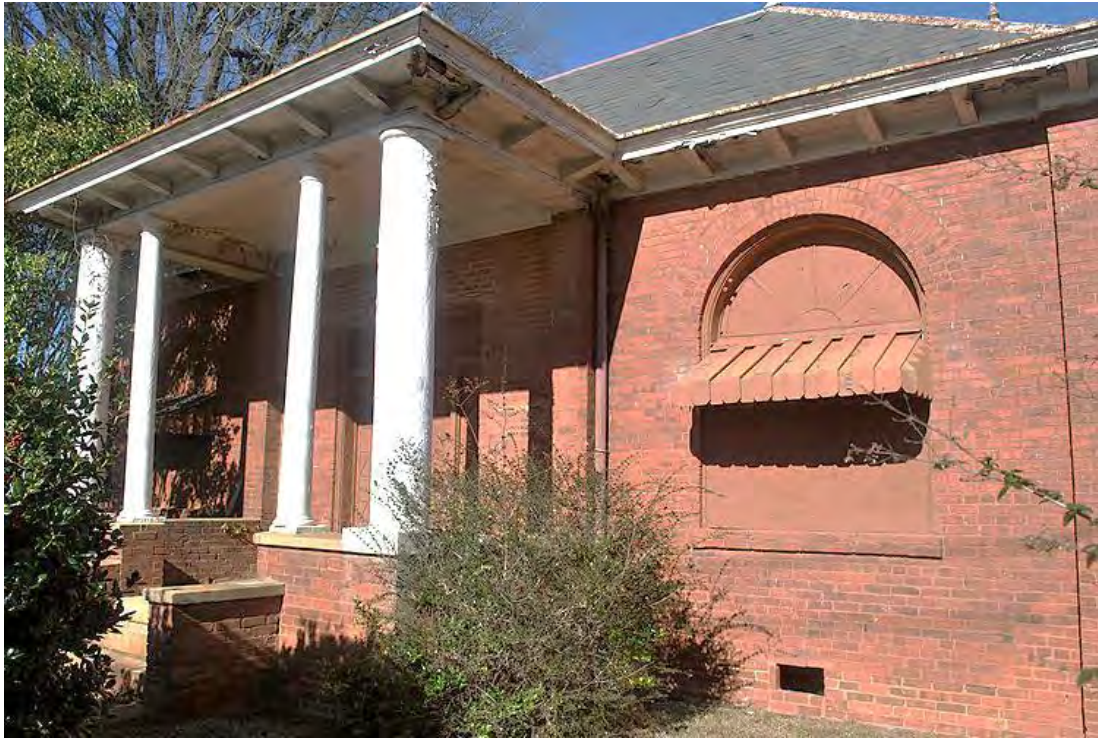
Lowell Cotton Mills, Mill Office, Façade, Looking Northwest.
