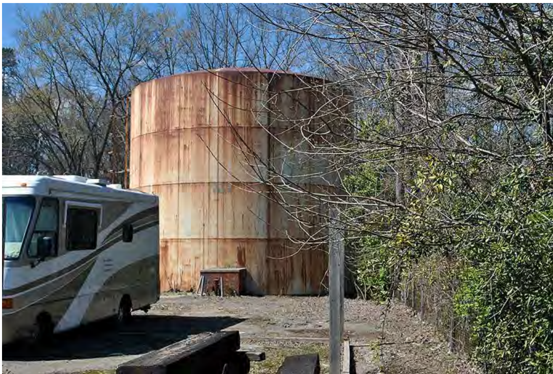
Modena Cotton Mills, Reservoir, Looking West.
