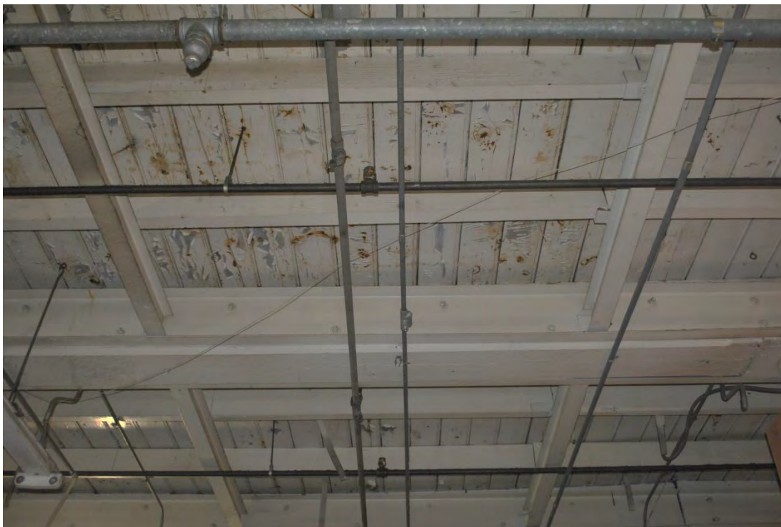
Modena Cotton Mills, Mill No. 2, Interior, Main Manufacturing Room, Ceiling.
