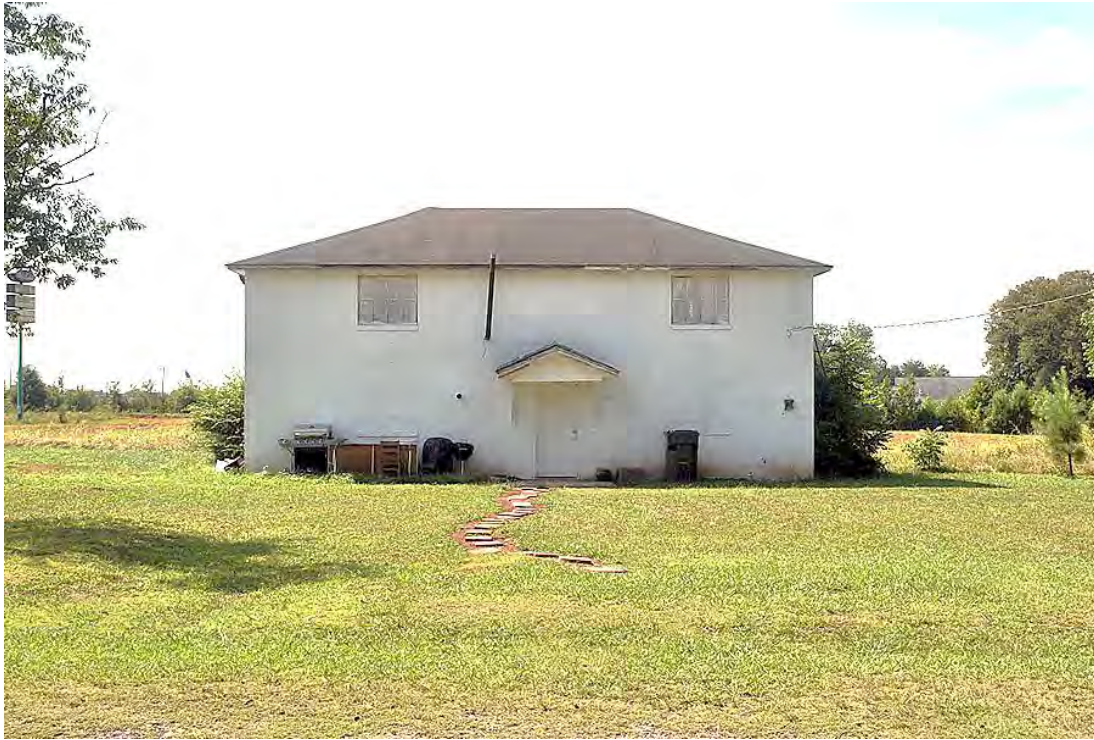
Hiram Masonic Lodge No. 22, Façade (North Elevation) Looking South from Wrights Chapel A.M.E. Zion Church.
