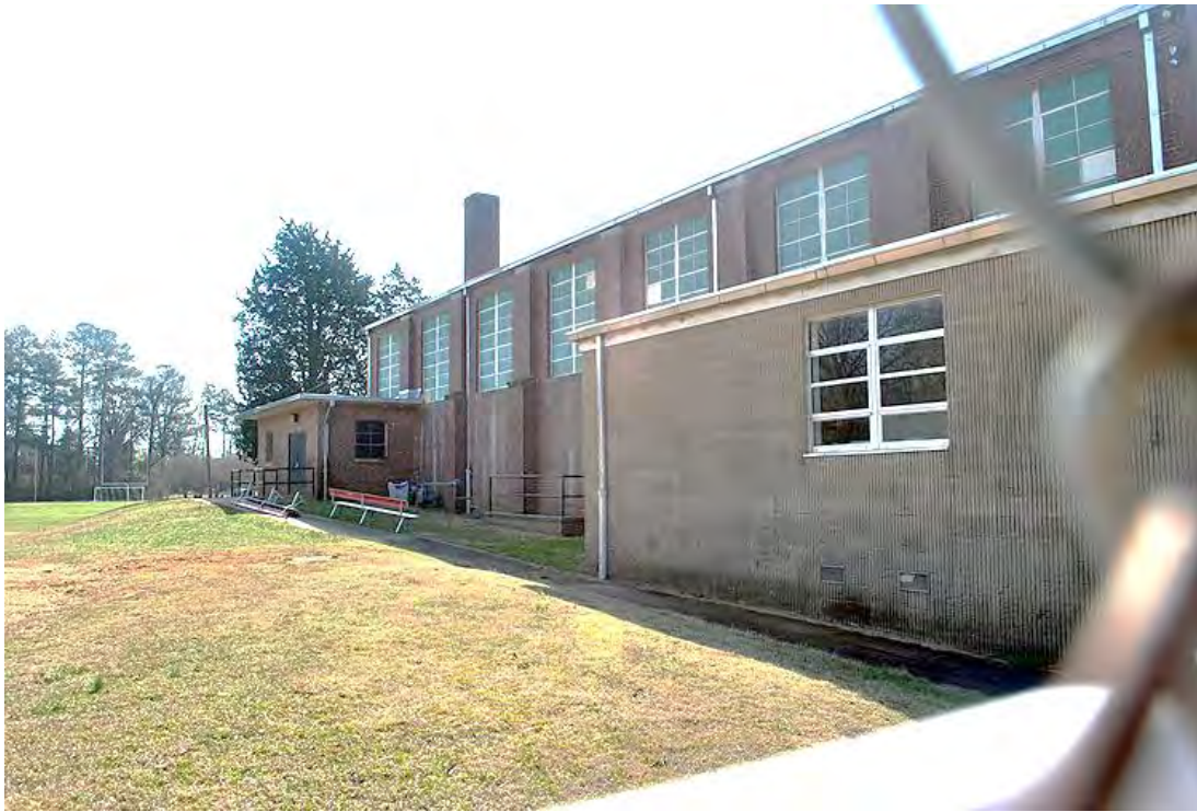
Holbrook High School, Gymnasium, North Elevation, Entrance Bay Addition, Looking East.
