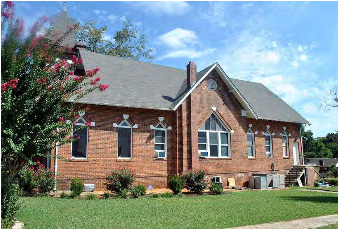
Wrights Chapel A.M.E. Zion Church, Side (South) Elevation, Looking Northeast.
