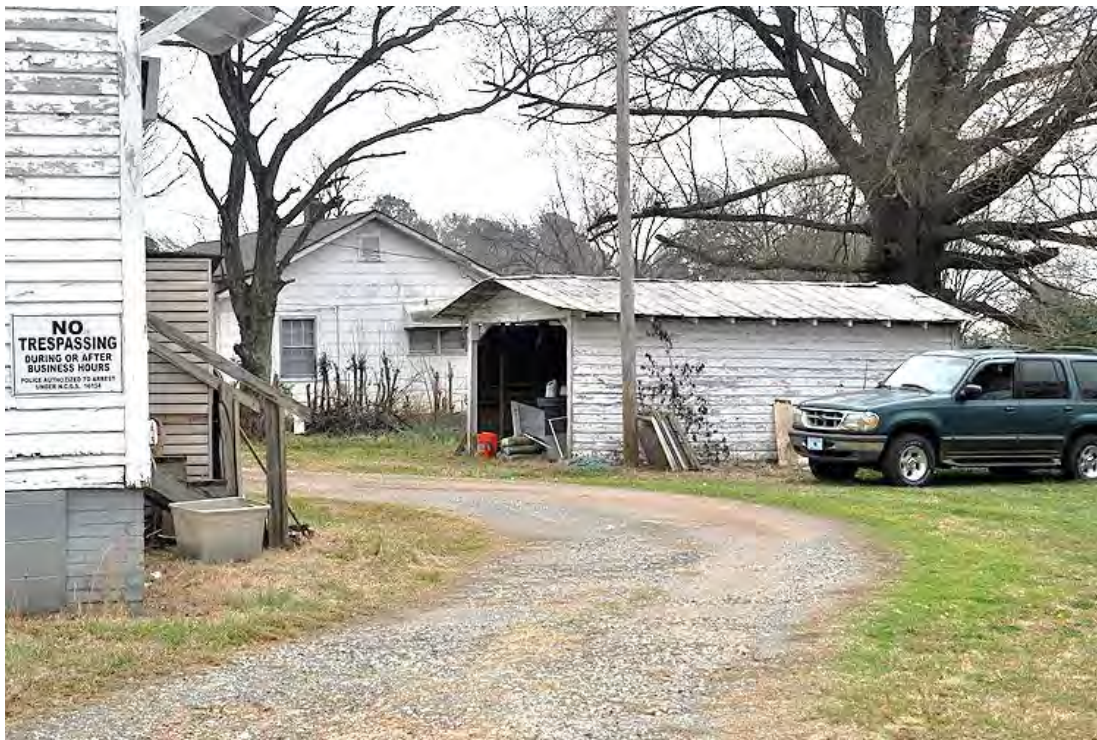
Nipper House and Store, Garage, Looking Southeast.
