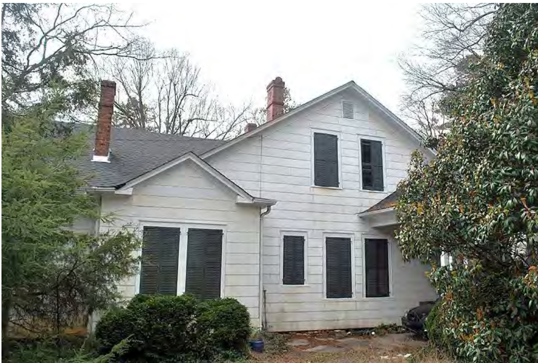
Paul P. and Virginia R. Murphy House, Side (North) Elevation, Looking South.
